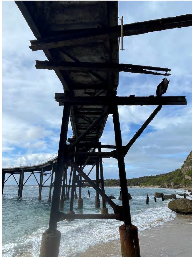
Figure 27 – Cantilever Beams to be Removed
