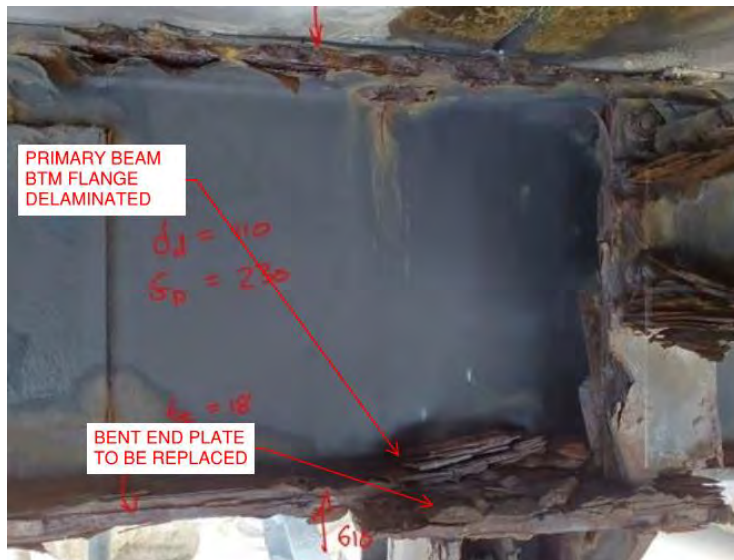
Figure 39 - Primary Beam to Bent Connection, Deck Type DC
