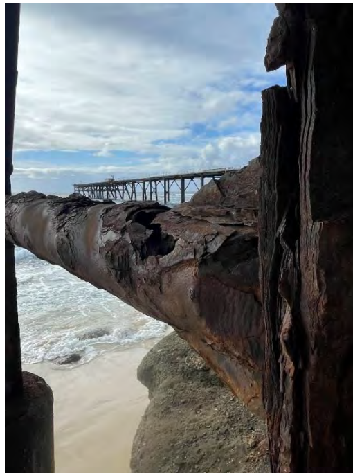
Figure 25 - CHS Horizontal Tie Bracing with Heavy Corrosion, Typical of Bents 18-28
