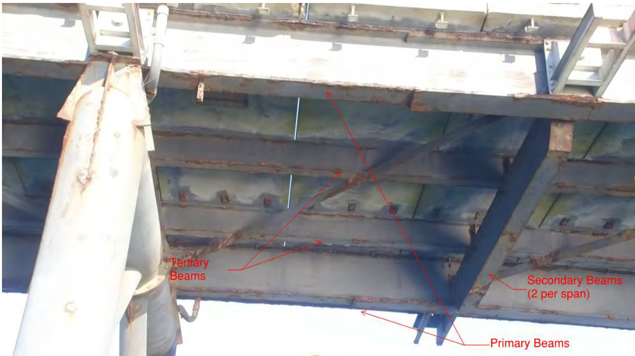
Figure 2 - Primary, secondary and tertiary beams
