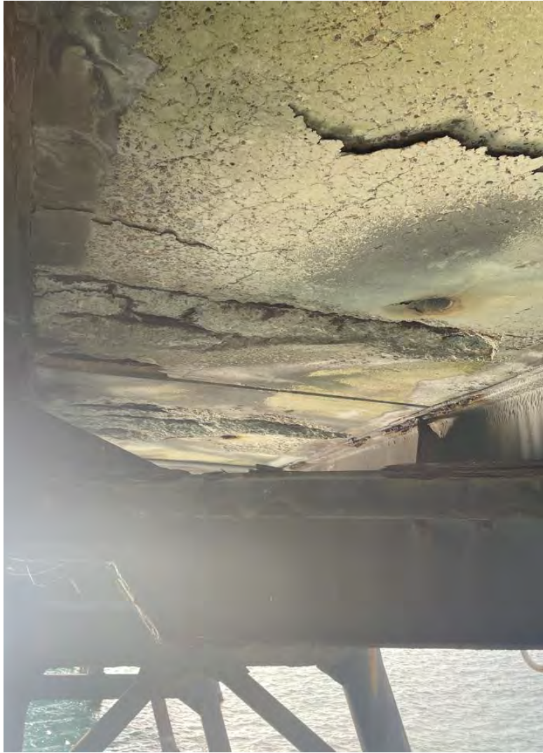
Figure 45 - Precast Panels Showing Deterioration with Reinforcement Exposed, Deck Type DB
