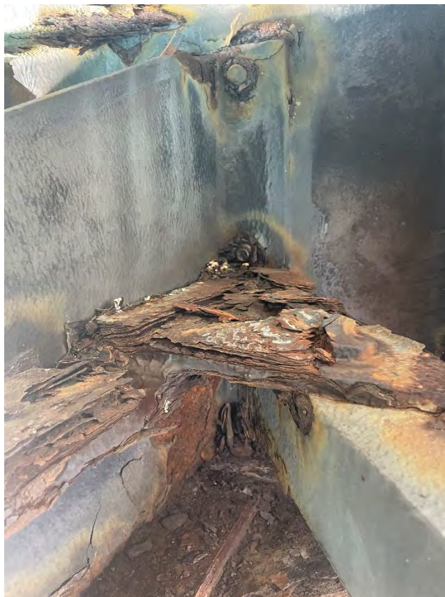
Figure 16 – Connection Between Plan Bracing, Secondary Beam and Primary Beam, Deck Type DB
