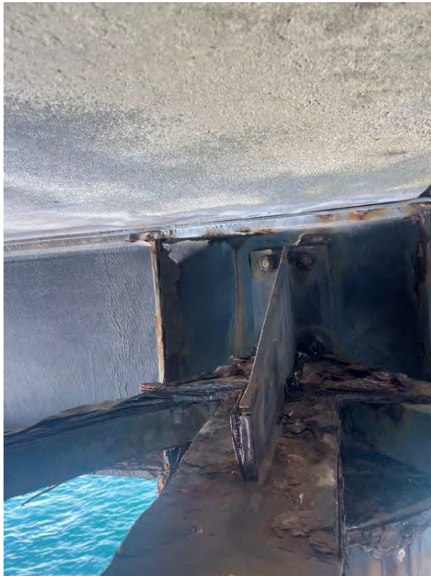
Figure 18 - Connection Between Secondary Beam and Primary Beam, Deck Type DA1
