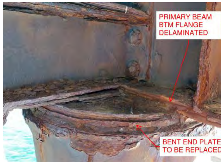
Figure 34 - Primary Beam to Bent Connection, Deck Type DA2
