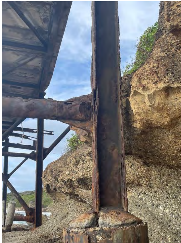
Figure 22 - 310 UC Column, Typical of Bents 18-28
