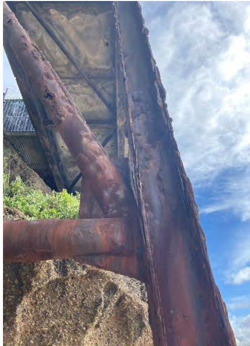
Figure 24 – CHS Vertical Bracing with Heavy Corrosion, Typical of Bents 18-28
