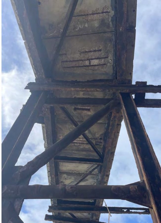
Figure 44 - Precast Panels Showing Deterioration with Reinforcement Exposed, Deck Type DC
