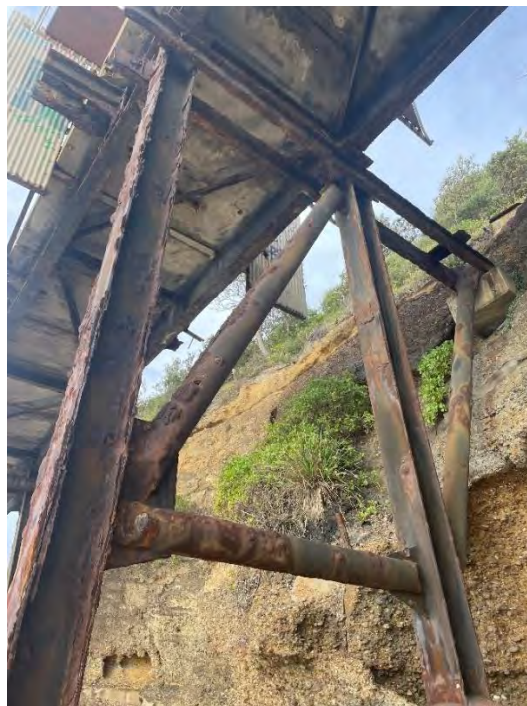
Figure 9 - Bents 24 to 28, typical inner Bent framing
