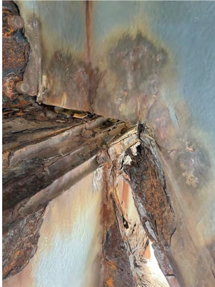
Figure 17 – Connection Between Secondary Beam and Primary Beam, Deck Type DA1
