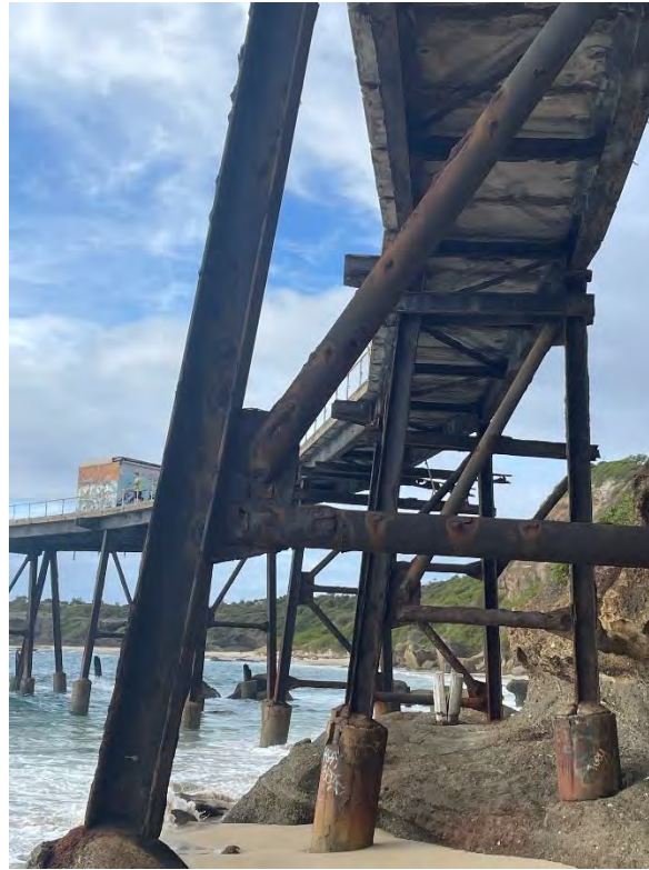
Figure 10 - Bents 24 to 28, typical inner Bent framing
