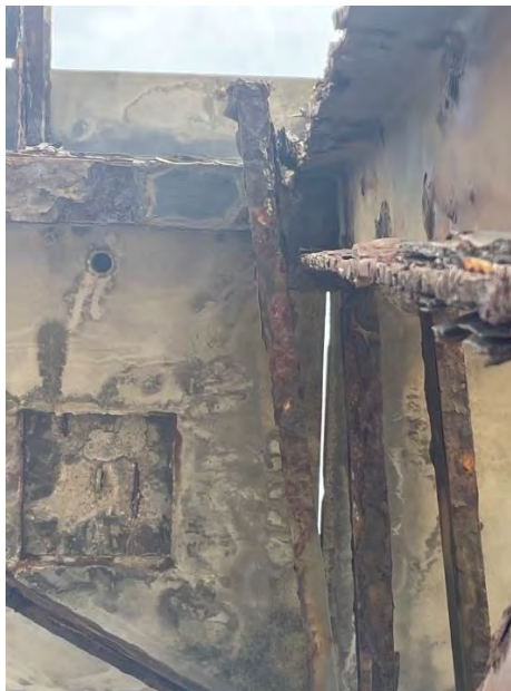
Figure 43 – Back-to-Back PFC, Visibly Detached from UC Columns, Typical of Bents 18-28
