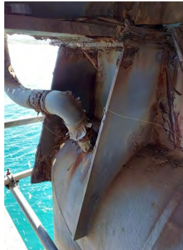
CONNECTION DETAIL - PRIMARY BEAM TO BENT
