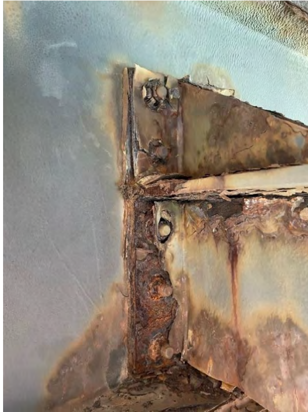
Figure 18 - Connection Between Secondary Beam and Primary Beam, Deck Type DA1
