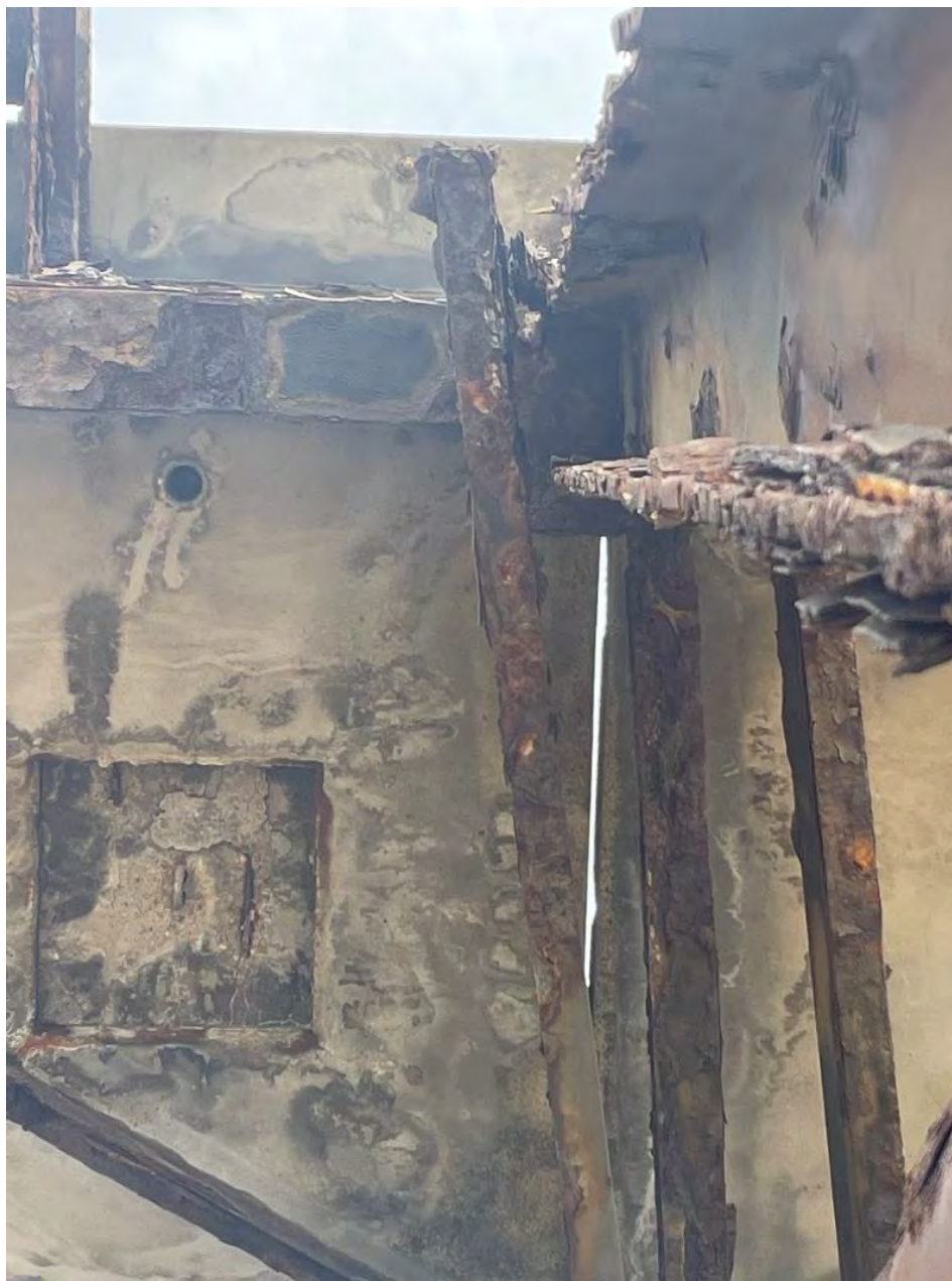
Figure 26 – Back-to-Back PFC, Visibly Detached from UC Columns, Typical of Bents 18-28
