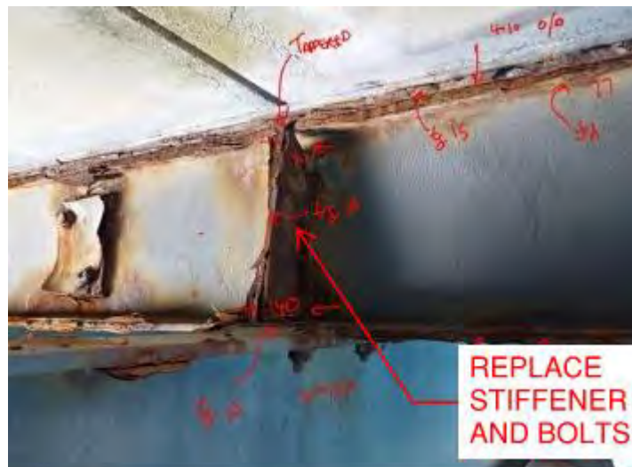
Figure 33 – Tertiary Beam to Secondary Beam Connection, Typical of Deck Type DA1
