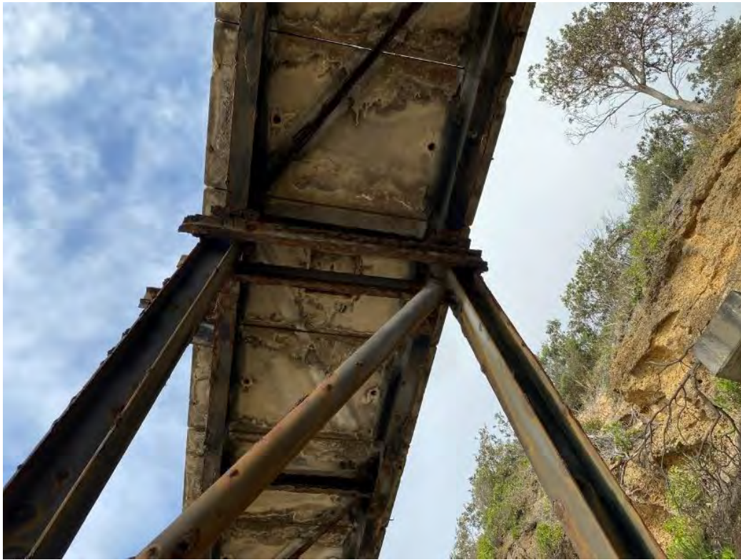
Figure 23 – Plan Bracing Missing Beneath Typical Deck Type DC
