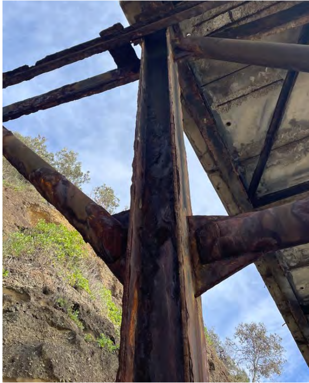
Figure 21 - 310 UC Column, Typical of Bents 18-28
