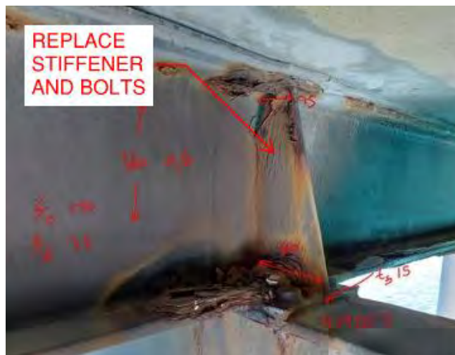
Figure 36 - Tertiary Beam to Secondary Beam Connection, Typical of Deck Type DA2
