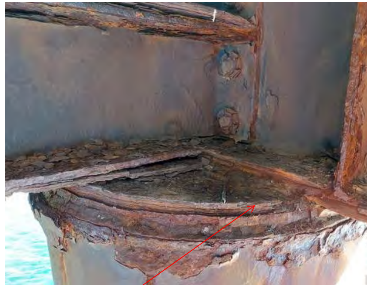
CONNECTION DETAIL - PRIMARY BEAM TO BENT
