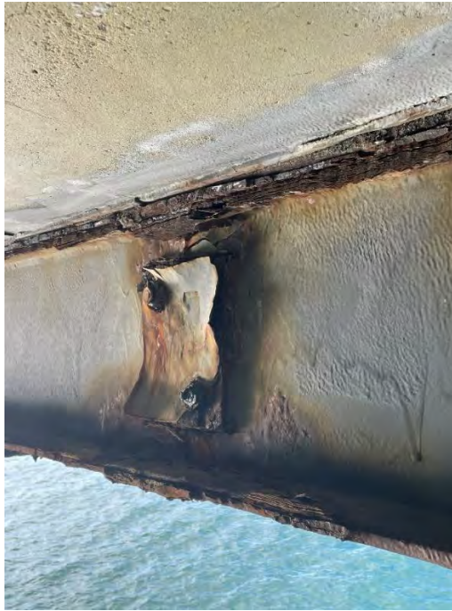
Figure 20 – Primary Beam Splice, Deck Type DB
