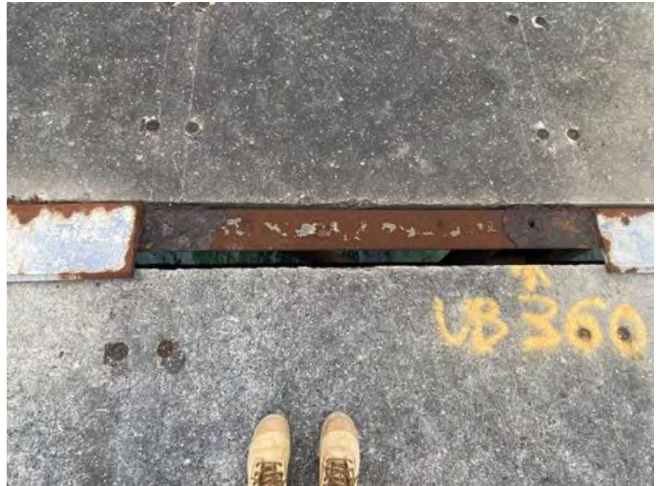
Figure 8 - Bent 17 movement joint
