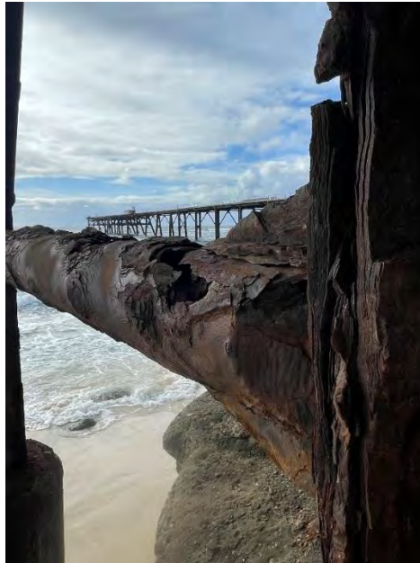
Figure 42 – CHS Tie Bracing Member, Typical of Bents 18-28
