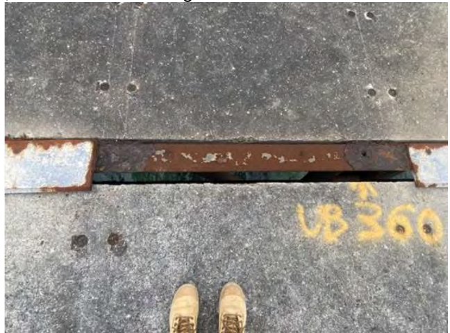
Figure 41 - Bent 17 movement joint
