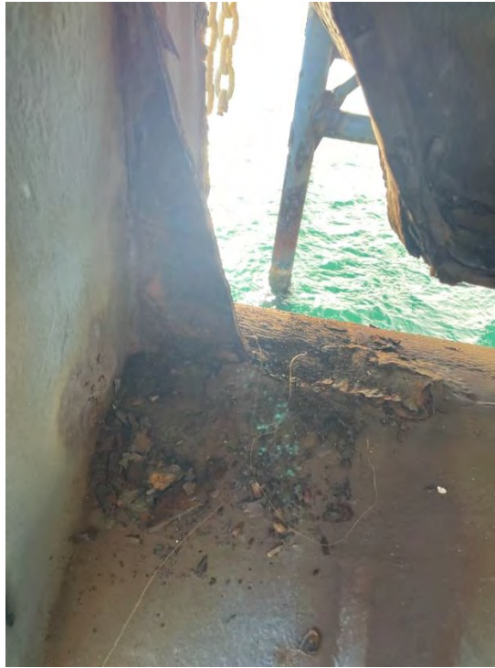
Figure 14 – CHS Tie Brace to CHS Column Connection
