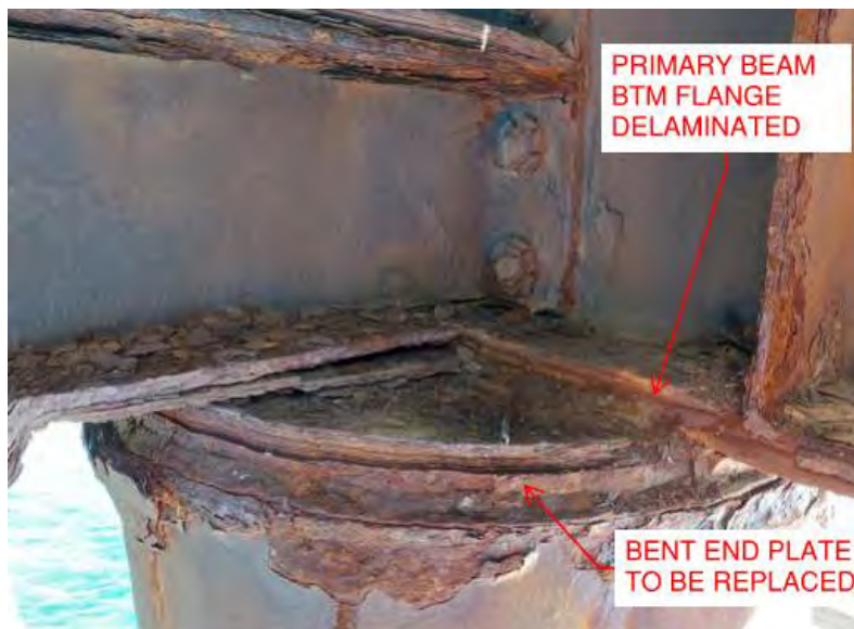
Figure 37 - Primary Beam to Bent Connection, Deck Type DB
