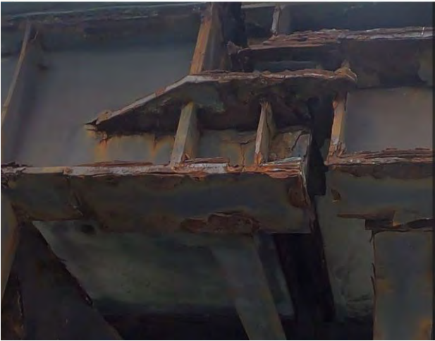
Figure 7 - Bent 17 Movement Joint
