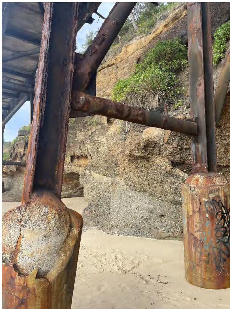
Figure 28 – Concrete Encasement for Corrosion Protection around UC Columns, Typical of Bents 18-28
