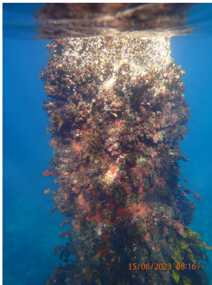
Photo 15: Pile 3. Before Clean. Underwater
