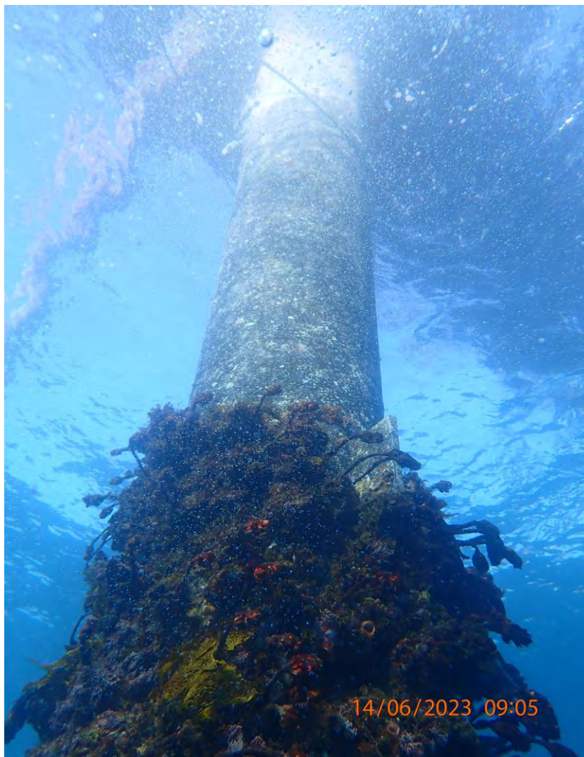
Photo 2: Pile 1. After Cleaning.
