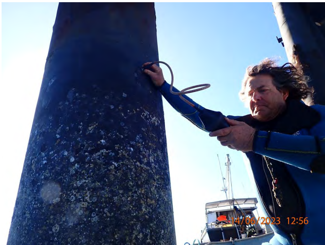
Photo 11: Pile 2. Testing High Water Mark.
