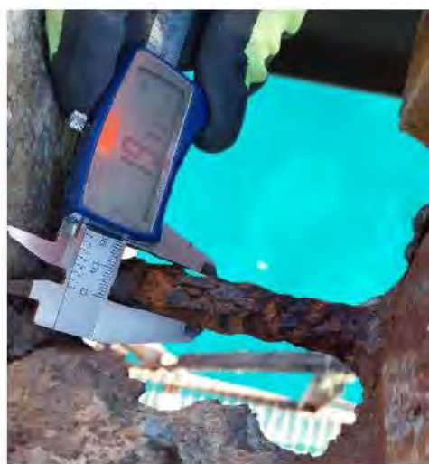
Figure 2: Exposed reinforcement
