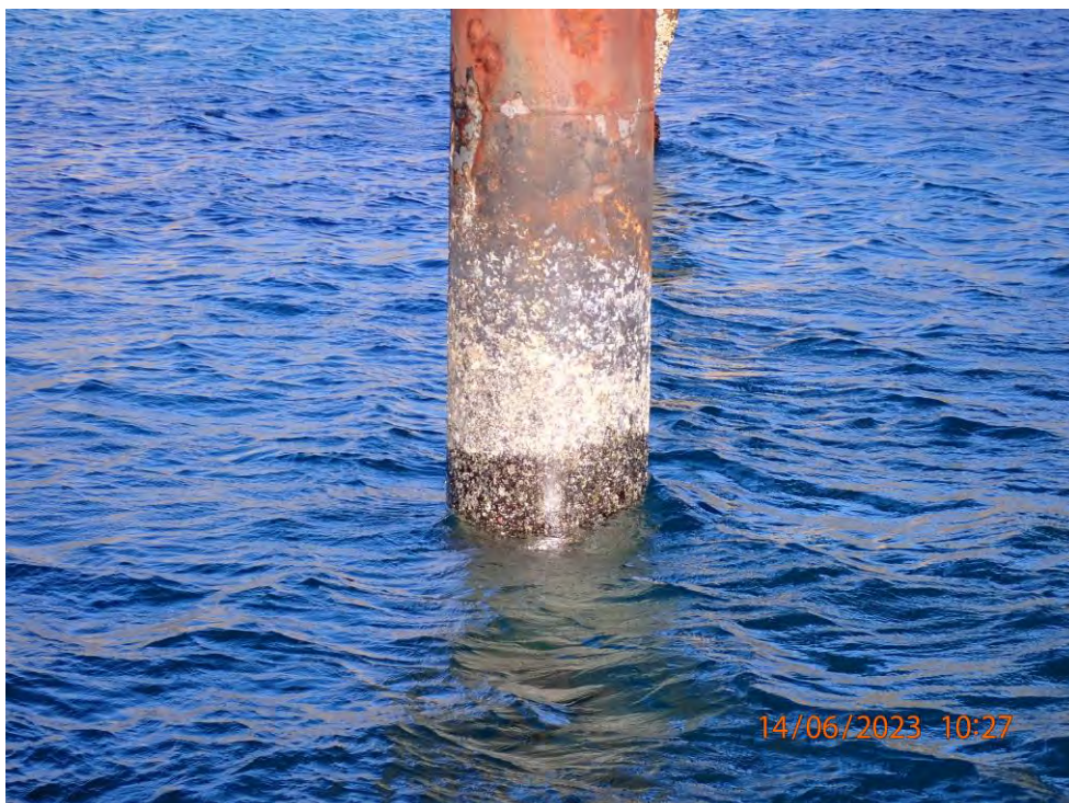
Photo 9: Pile 2. After Cleaning. High Water Mark.
