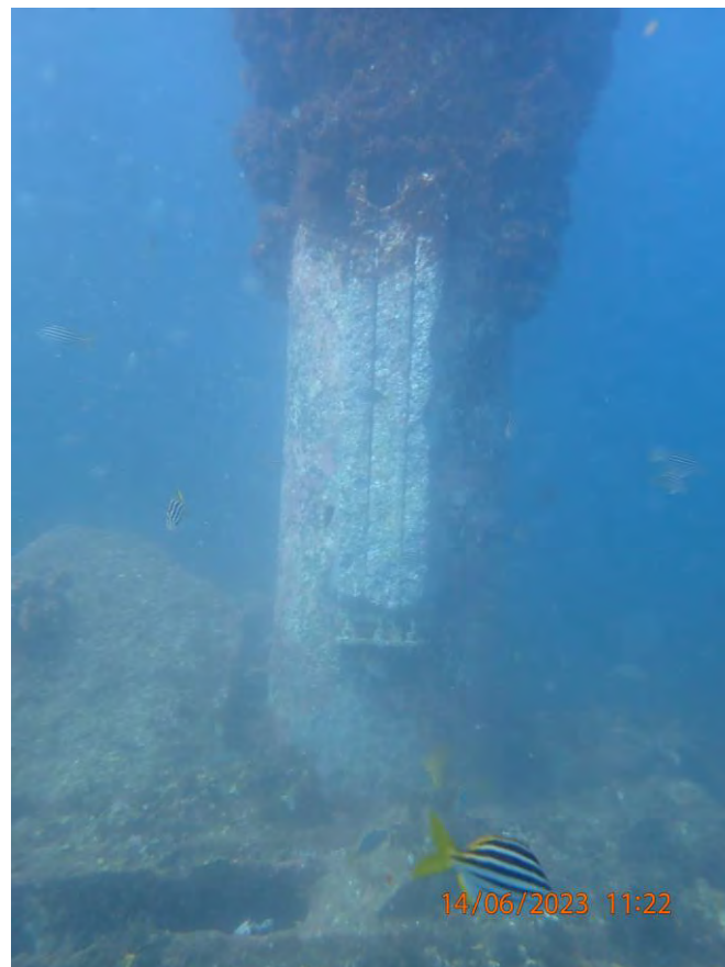
Photo 13: Pile 2 Anode
