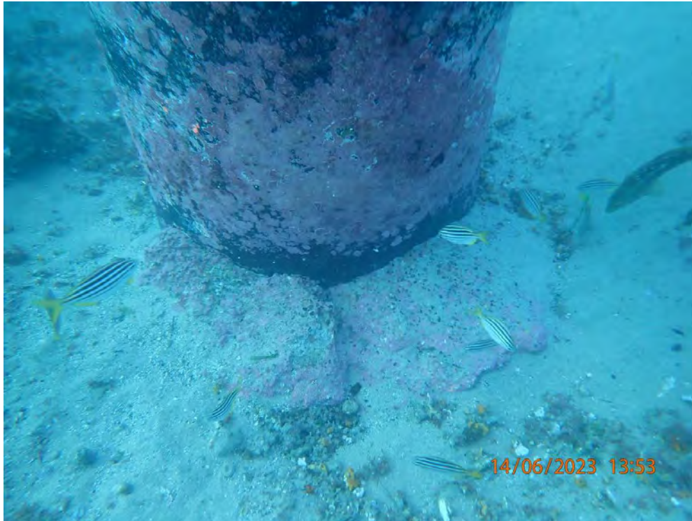
Photo 7: Pile 2. Before Cleaning. High Water Mark
