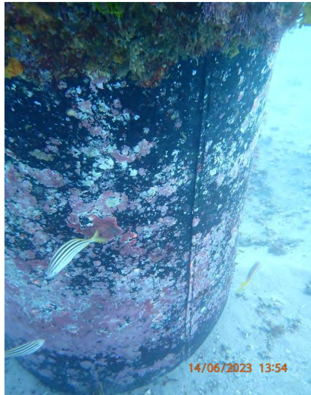
Photo 5: Pile 1 Plastic Wrap
