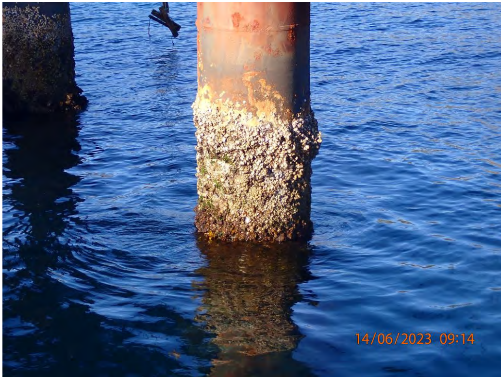
Photo 7: Pile 2. Before Cleaning. High Water Mark
