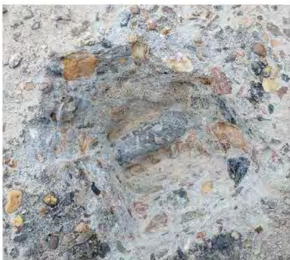
Figure 1: Reinforcement breakout
