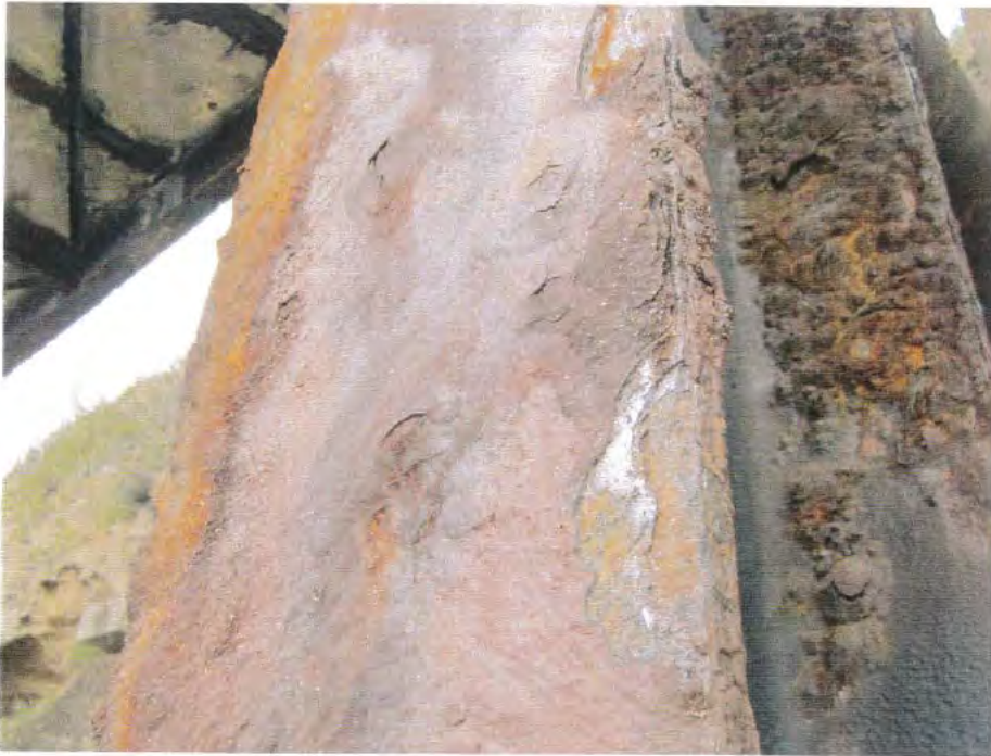
Photo 17. A detailed view of corrosion damage to both the inner and outer faces of a Bent leg.
