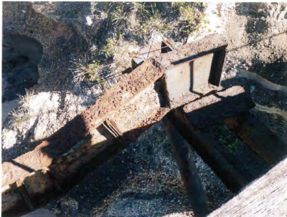
Photo 6. A detailed view of corrosion damage to ancilliary structure connected to Bent 24.
