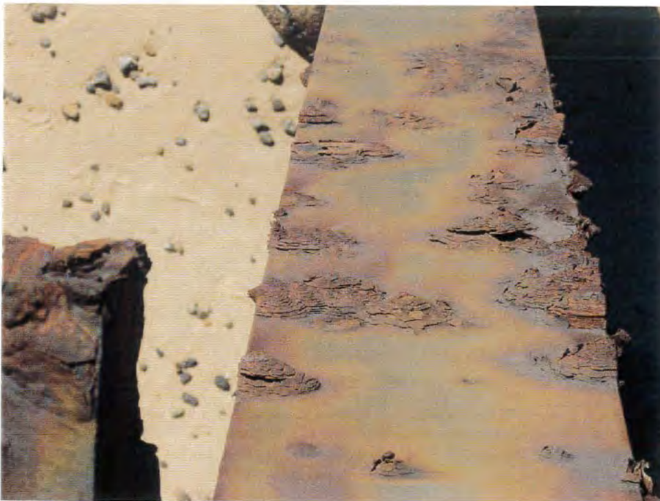
Photo 2. A detailed view of corrosion on the face of a column Bent shown in Photo 1.
