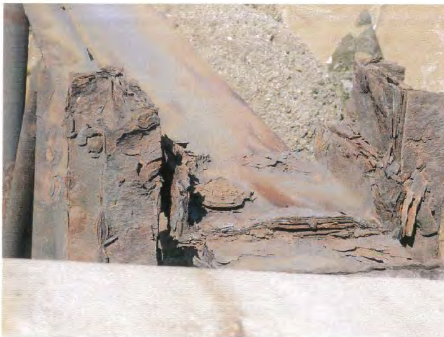
Photo 5. A detailed view of corrosion damage to the top of a Bent leg and the interconnecting PFC's shown in Photo 4. Note the failure of the welds between the PFC's and the leg.
