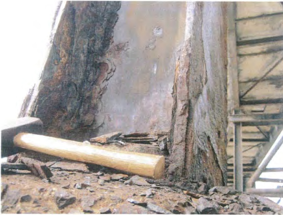
Photo 25. A detailed view of corrosion at the base of a Bent leg. Note the amount of rust scale.
