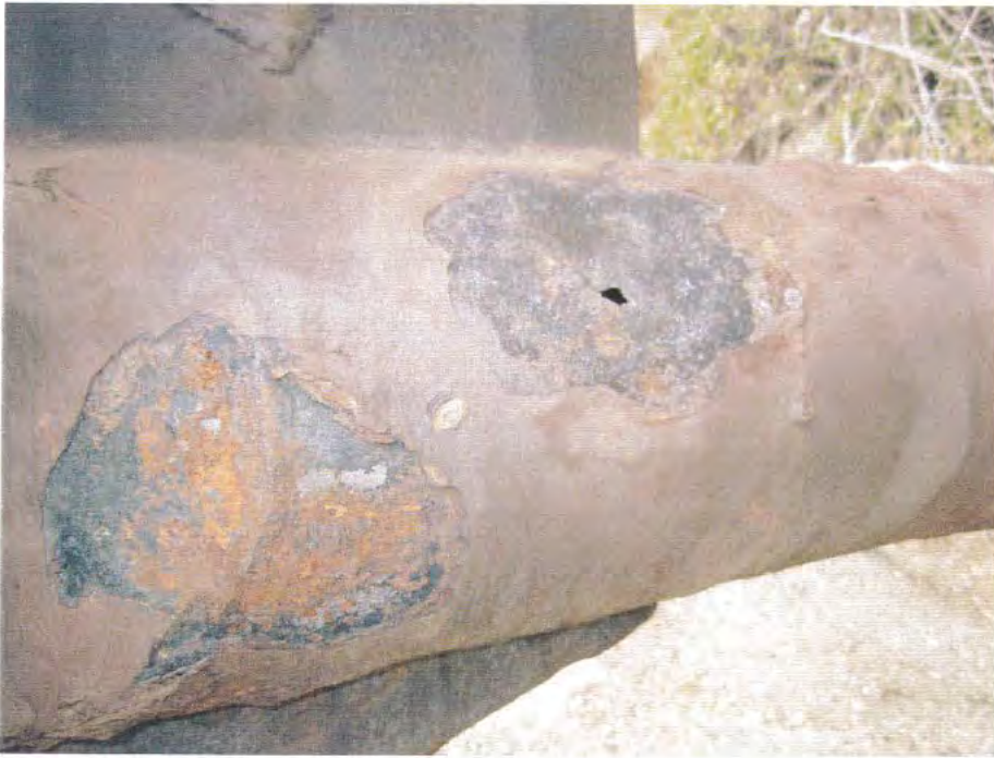
Photo 21. A detailed view of corrosion damage Bent brace member.
