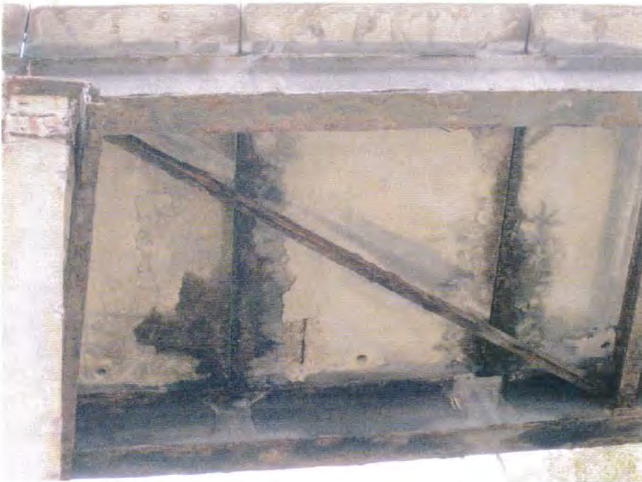
Photo 28. A detailed view of the soffit of a deck section. Note the corrosion to the reinforcing, deck brace, primary beam flanges, inter-leg PFC and the failed weld connection between the PFC and leg.
