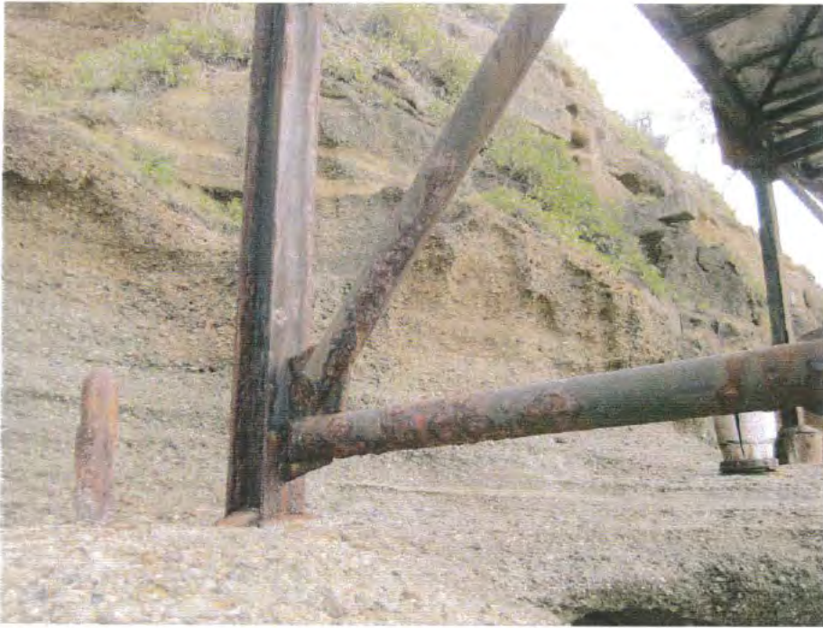
Photo 29. A detailed view of corrosion damage to the base of a Bent. Note the damage to the connection plate.
