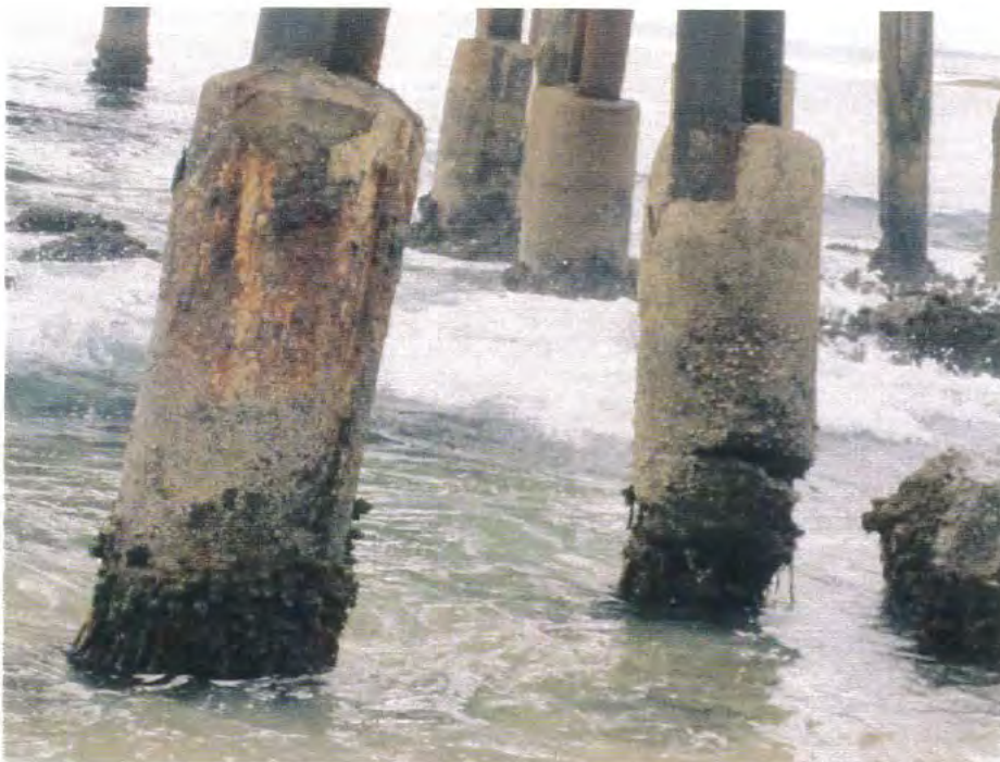
Photo 32. A detailed view of the base of a steel leg. Note the leg is supported on a timber pile with a connection that appears to be a damaged concrete encasement.
