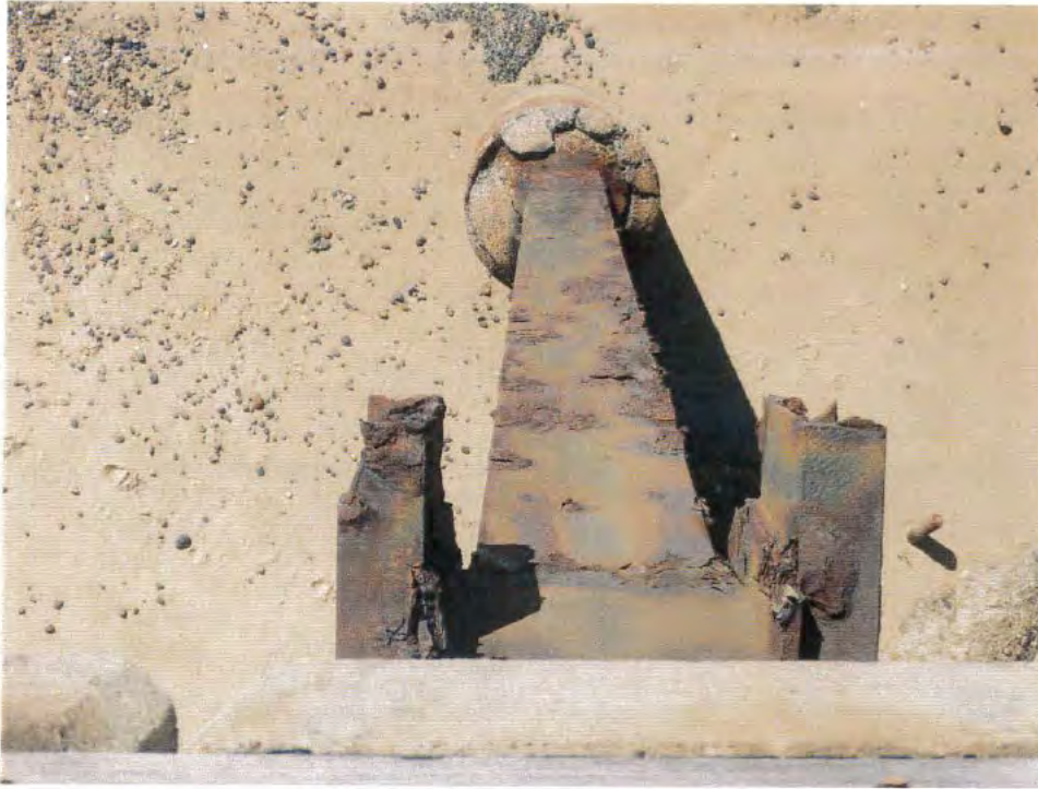
Photo 1. A view down the outer leg of a Bent. Note the overall corrosion and the corrosion damage to the interconnecting PFC's and their welded connections.
