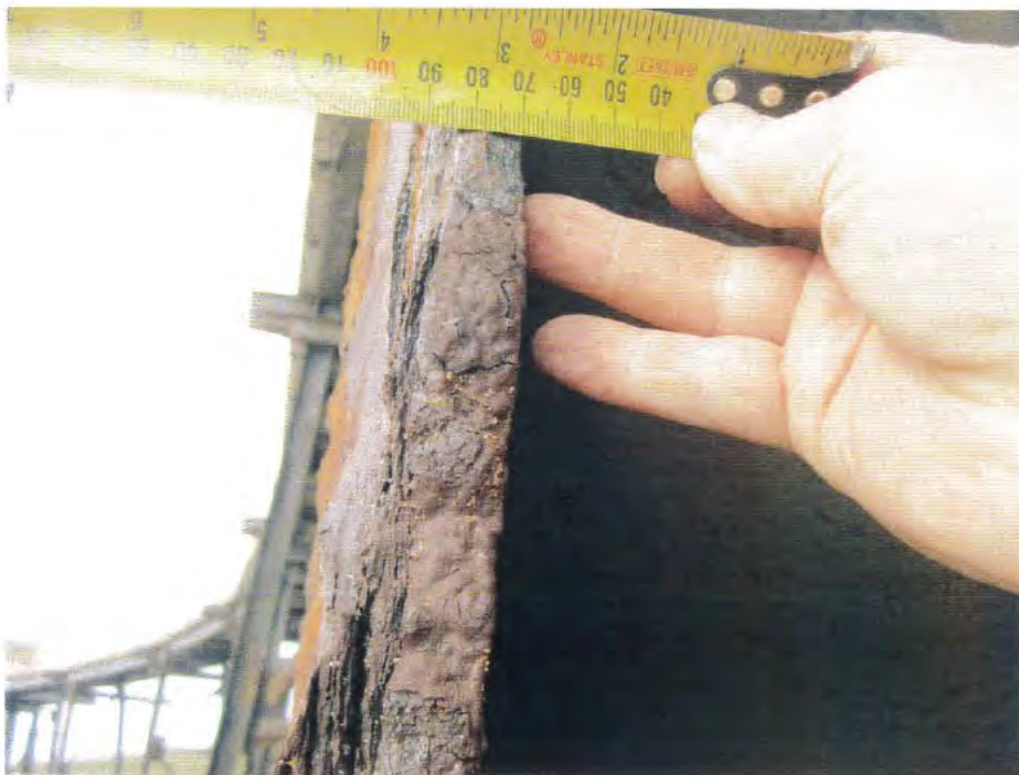
Photo 16. A detailed view of a corrosion reduced Bent leg flange. Note: the flange thickness was originally 18.5mm.
