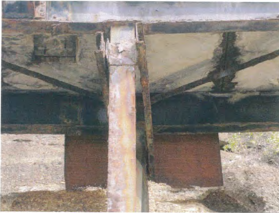
Photo 31. A detailed view of the top of Photo 30. Note the corrosion damage to the steelwork and in particular the separation of the left hand PFC from the leg due to weld failure from corrosion.
