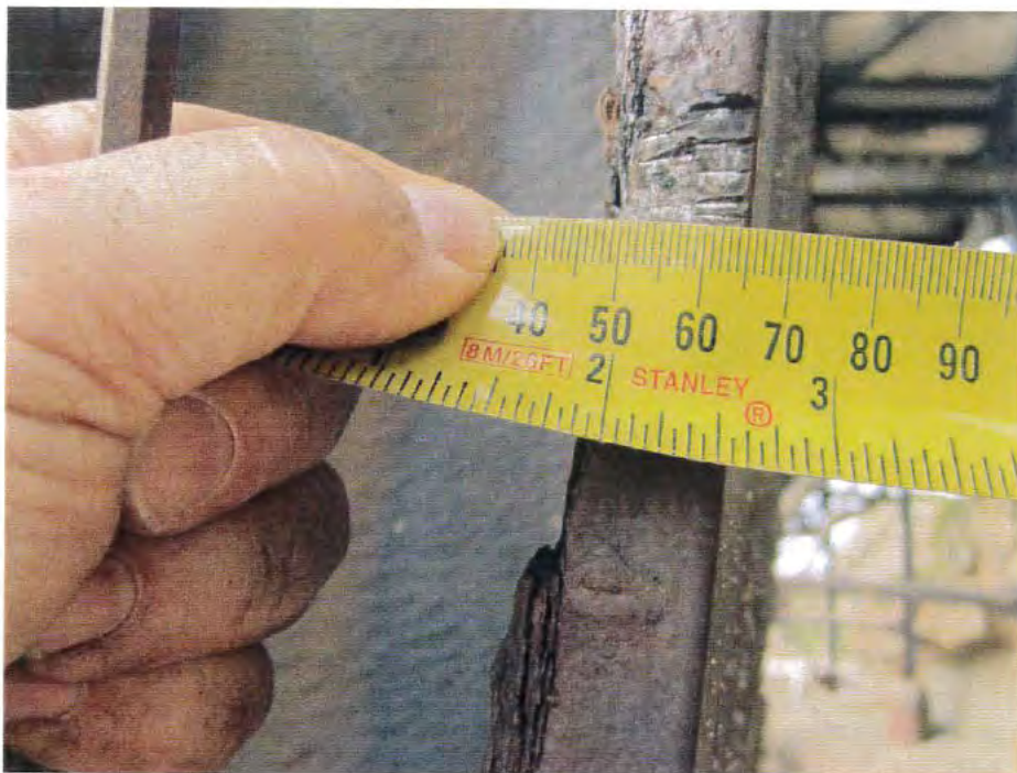
Photo 18. A detailed view of a corrosion reduced Bent leg. Note the flange thickness was originally 18.5mm.
