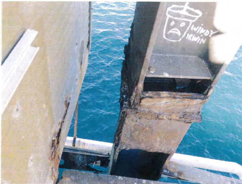
Photo 14. A detailed view of corrosion damage to a derrick near bent 4. Note: the concentration of rust around the heavily welded sections.
