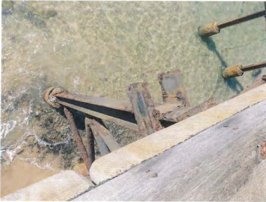
Photo 7. A detailed view down the length of a Bent leg. Note the damage to the concrete encasement and the PFC ties that run between the legs of the bent.
