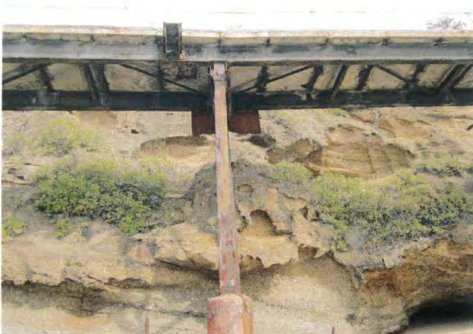
Photo 30. A view of the outer leg of the Bent shown in Photo 29. Note the rust staining on the concrete encasement.
