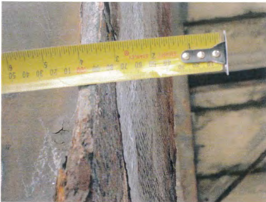
Photo 24. A view of corrosion reduced flange thickness. The original thickness was 18.5mm and is now 12mm.
