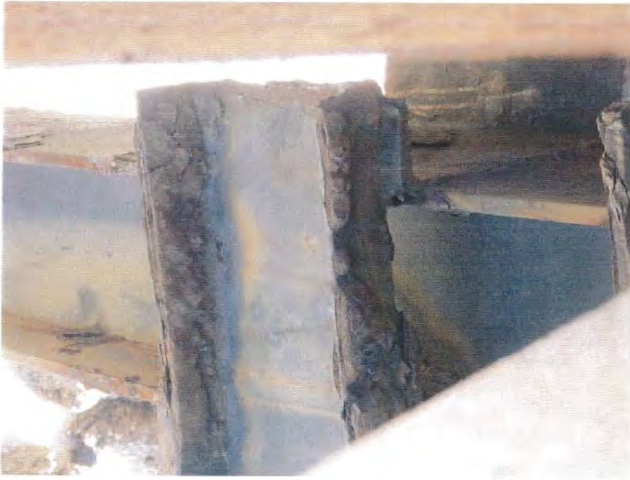
Photo 3. A detailed view of corrosion damage to the top of a Bent column.
