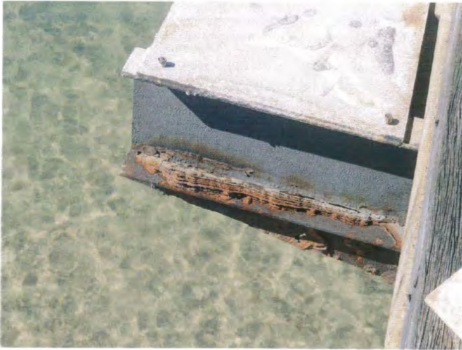
Photo 9. A detailed view of corrosion to the bottom flanges of PFC tie members that connect the Bent legs immediately under the primary deck beams.
