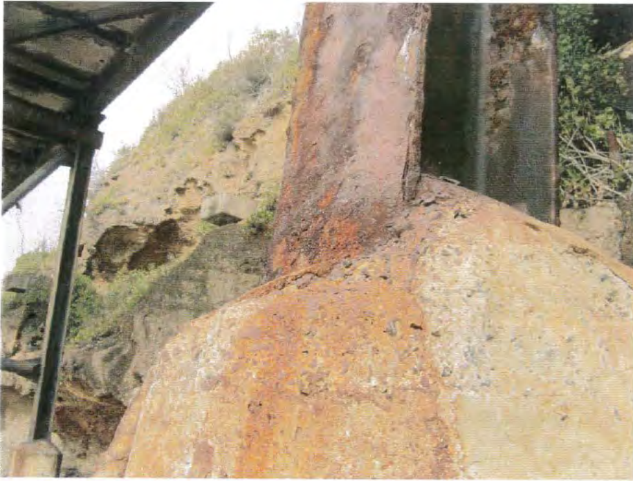
Photo 19. A detailed view of the base of a Bent leg. Note the rust staining and the swelling of the flanges.
