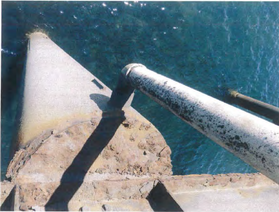
Photo 11. A typical view of corrosion on the CHS Bent leg cap plate. Note the corrosion of the primary beam flange.
