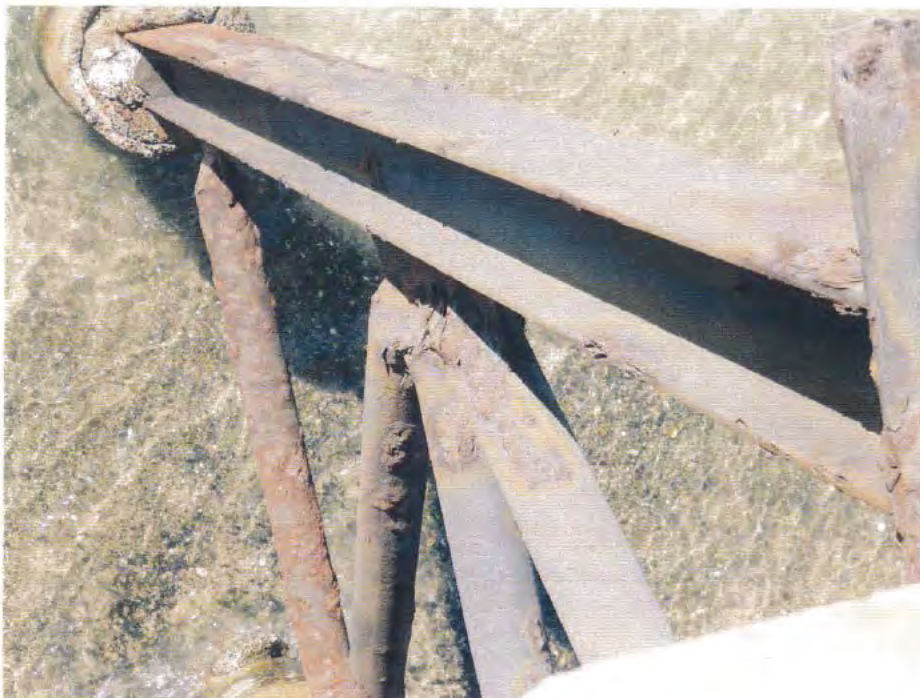
Photo 8. A detailed view of corrosion damage to the bracing members for the Bent shown in Photo 7.
