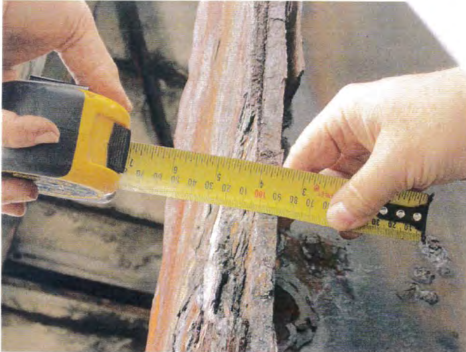
Photo 22. A detailed view of a corrosion reduced flange.
