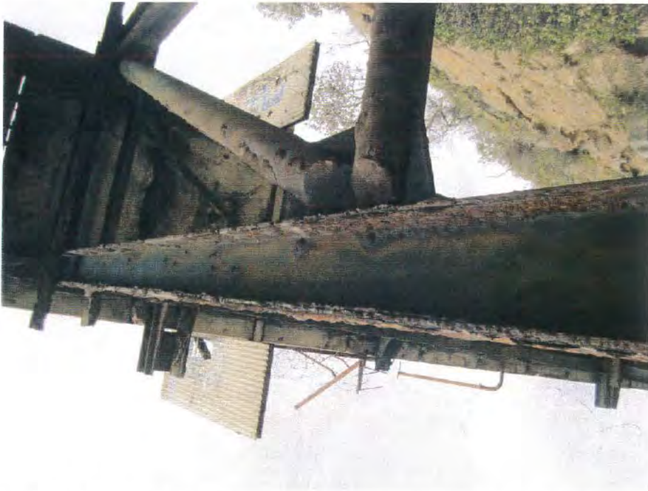
Photo 15. A detailed view of the outer leg of a Bent. Note the corrosion damage to the leg and brace members.
