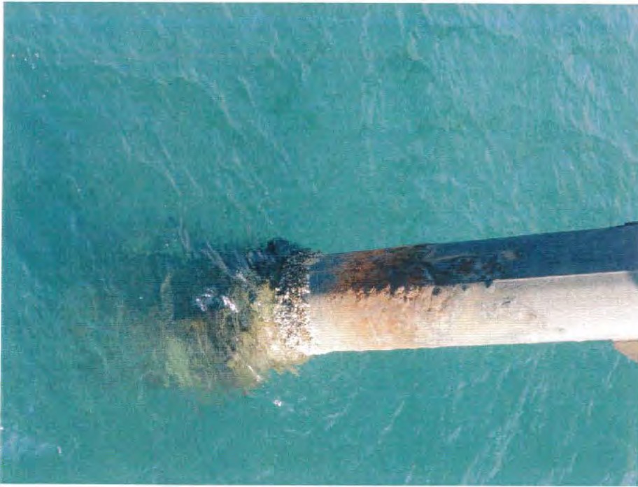
Photo 13. A typical view of corrosion at the base of a CHS Bent.
