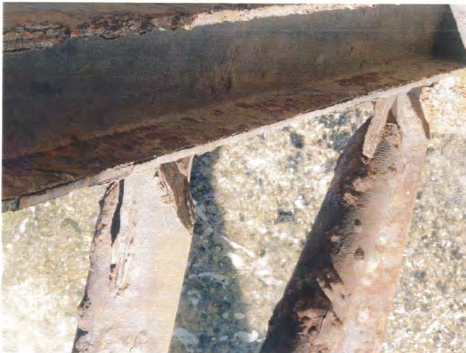
Photo 10. A detailed view of corrosion in the brace elements of a Bent frame.
