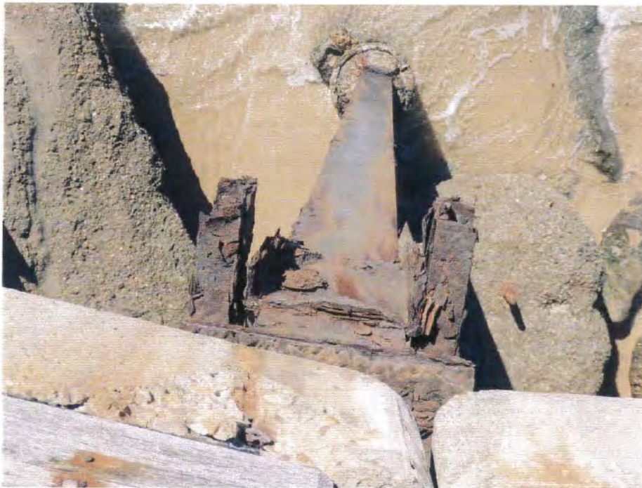
Photo 4. A detailed view of severe corrosion at the top of a Bent.
