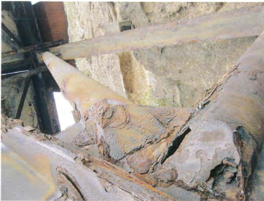
Photo 26. A detailed view of a corroded Bent bracing connection.
