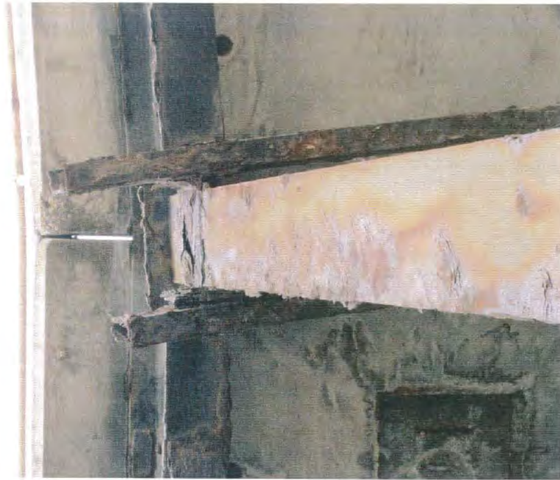
Photo 23. A detailed view of corrosion damage to the interconnecting PFC members. Note the failed welded connections between the PFC's and the leg.
