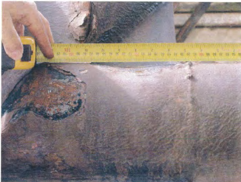
Photo 20. A detailed view of corrosion damage to a Bent brace member. Note the dent in the top of the member.
