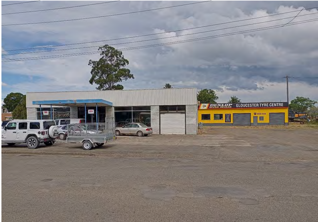
Photo 1: Looking south at the site from Denison Street (18 April 2024)
