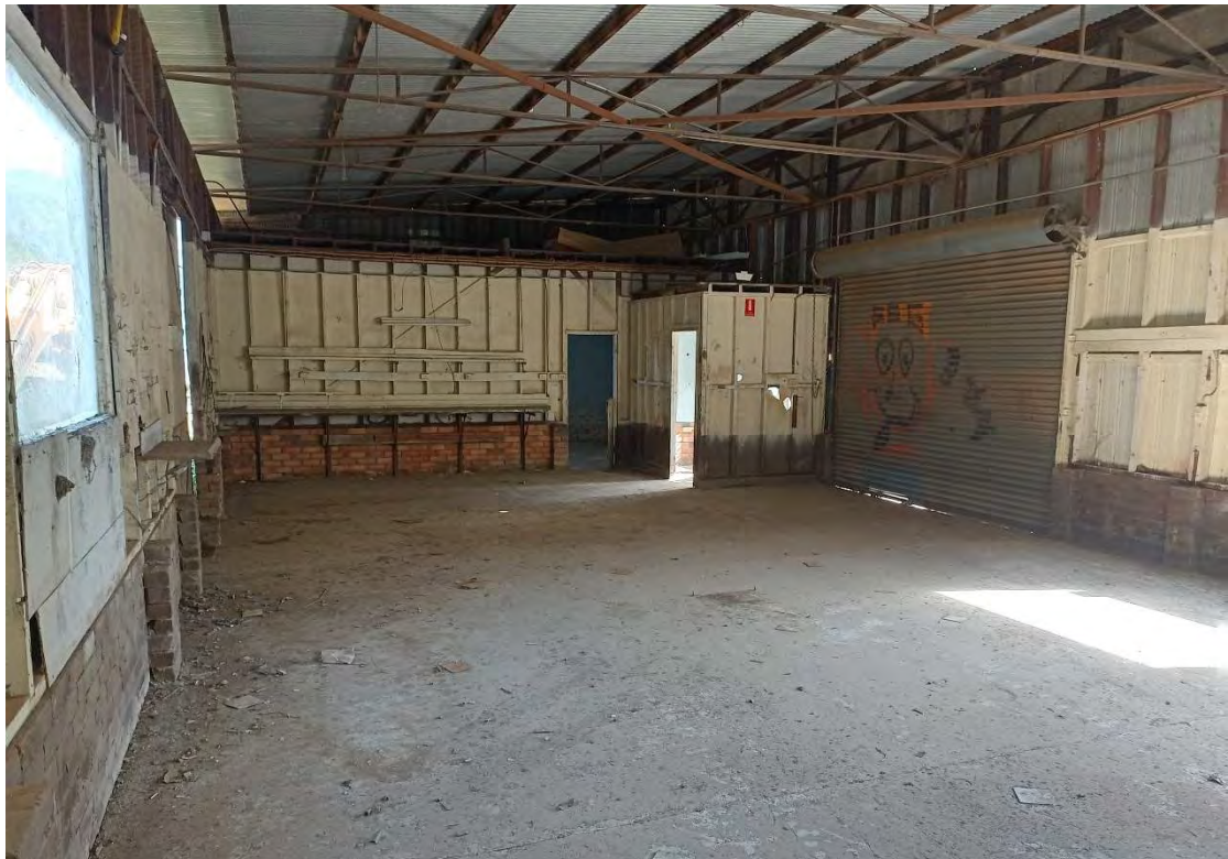
Photo 10: Looking west across former tyre workshop (18 April 2024)
