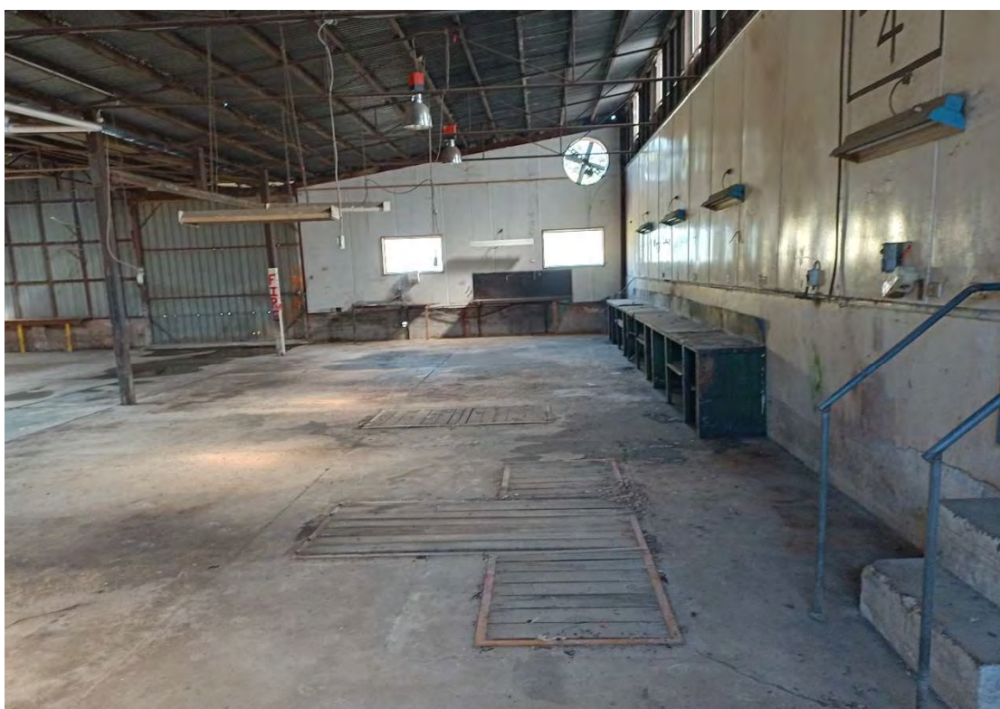
Photo 6: Looking east across former workshop. Possible inspection pits observed (18 April 2024)
