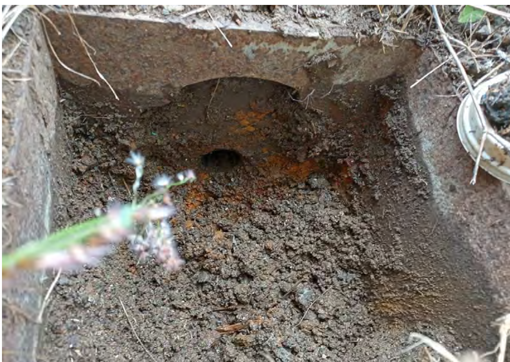
Photo 6: Drainage pipe within sump leading towards the creek adjacent the site (31 March 2025)
