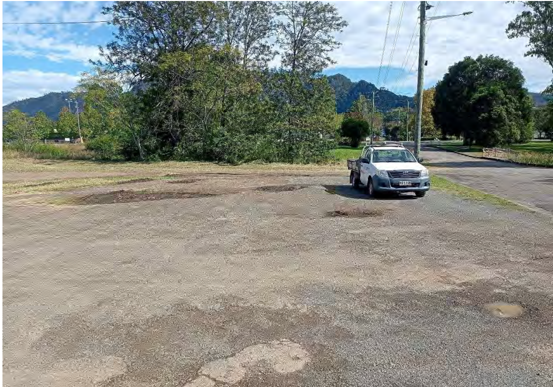
Photo 13: Looking west at the north western corner of the site (18 April 2024)
