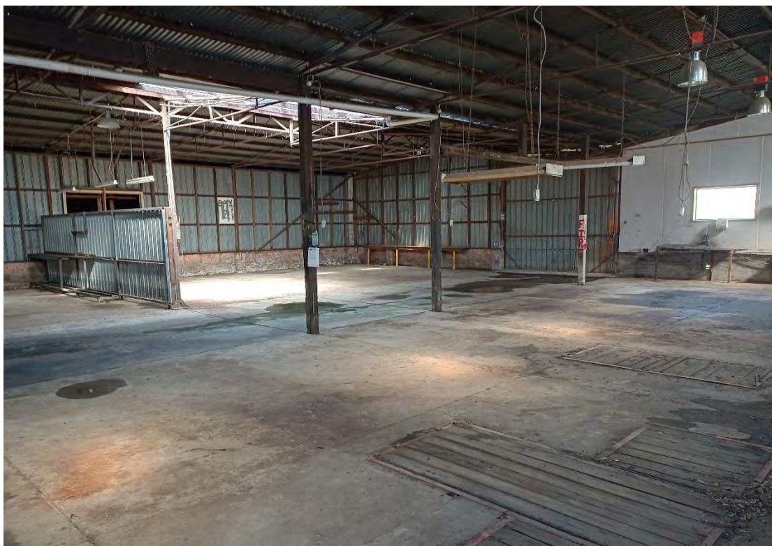
Photo 7: Looking across former workshop (18 April 2024)
