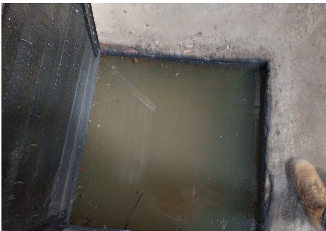
Photo 8: Inspection pit filled with water at the time of the initial inspection (18 April 2024)
