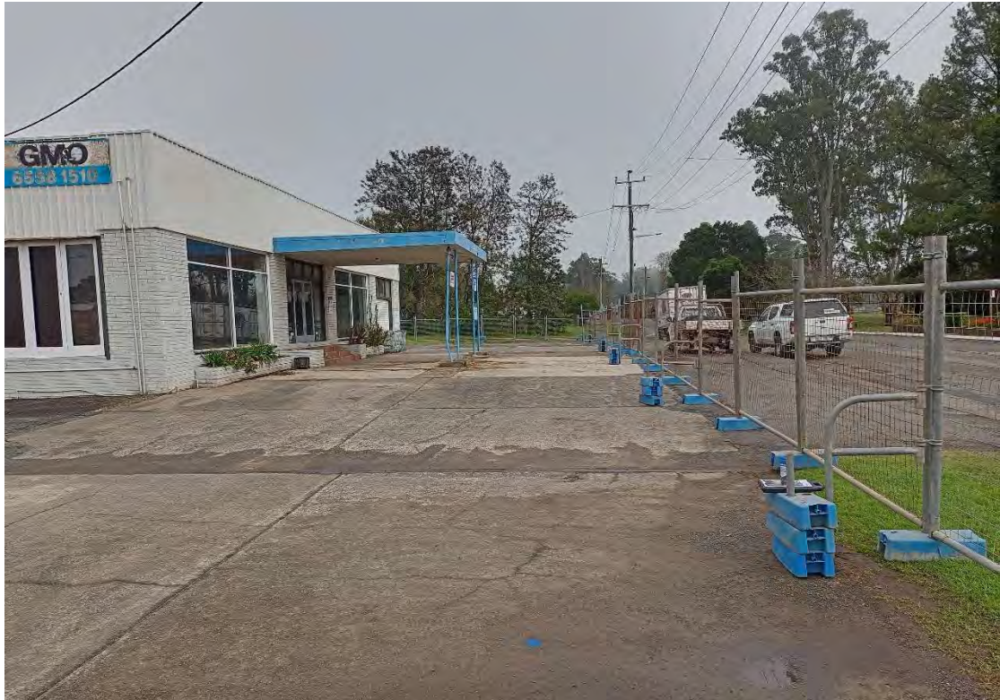
Photo 23: Looking along the northern boundary of the site at tank farm (6 June 2024)
