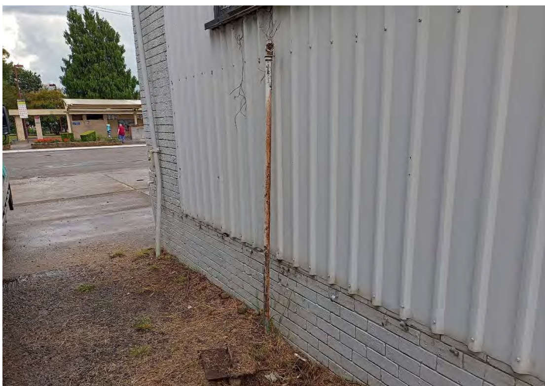
Photo 16: Waste sump and possible breath point for USTs in the northern portion of the site (18 April 2024)
