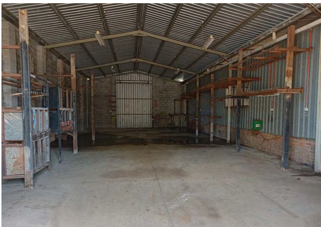
Photo 12: Looking west across shed (18 April 2024)
