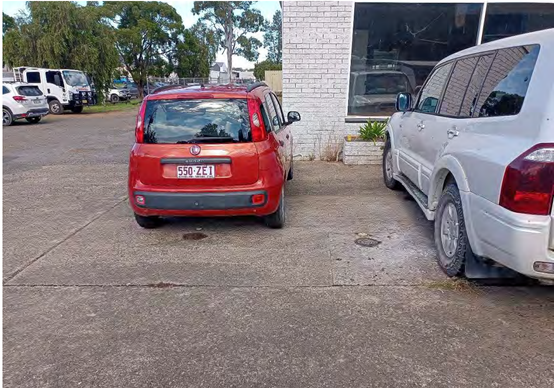
Photo 3: Fill points for two 4,500L unleaded USTs in north eastern portion of the site (18 April 2024)
