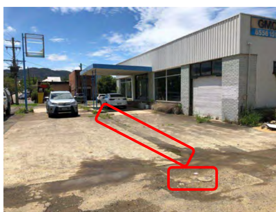
Looking east showing the front of the existing building. Two UST fill point are visible on the ground surface and what appears to be the location of the old fuel lines connecting the USTs to the bowsers (bound by red outlines).
