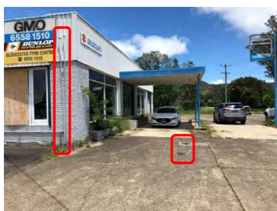
Looking west showing the front of the existing building which was a former machinery shop and service station. Two UST fill point are visible on the ground surface and two breathe pipes are shown on the outside of the building on the left (bound by red outlines).
