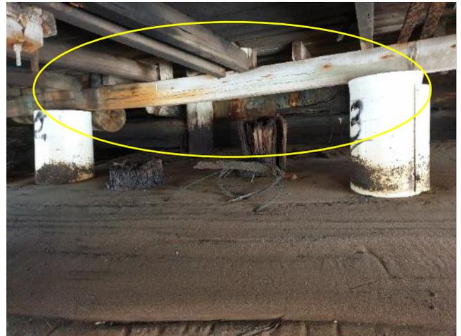
Photograph 23 shows timber joist has slipped off the bearer.
