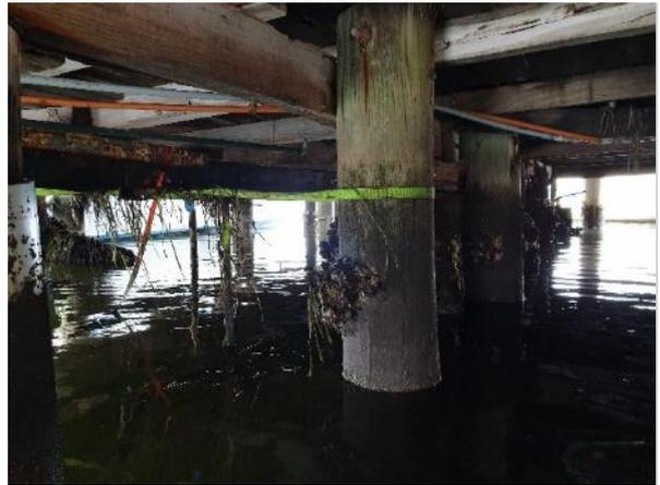
Photograph 2 shows an example of ratchet straps providing some form of support / tie-down / tension bracing to prevent separation in subfloor framing members.
