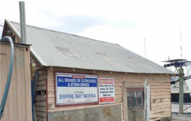
Photograph 47 shows the roof cladding above boat shed appears satisfactory.
