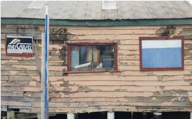
Photograph 61 shows an example where 2x windows have been covered over, along with centre window in a 'weathered' state.
