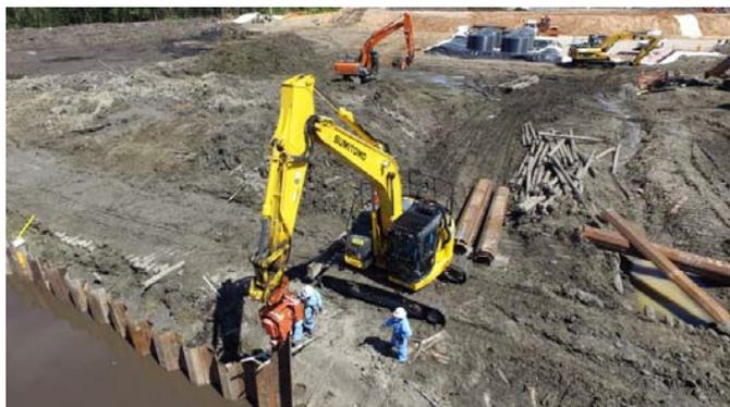
**Installing a sheet pile wall to hold back the wetland water**
