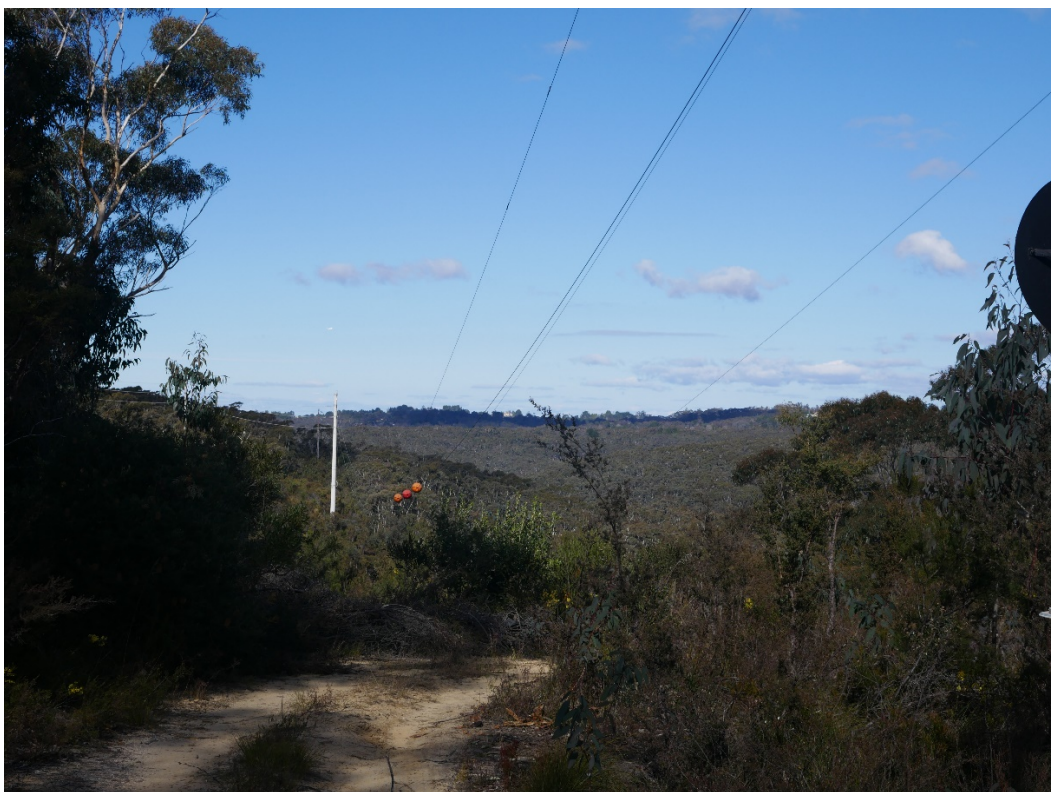
66 kV transmission line 100 m west of runway YKAT 06/24
