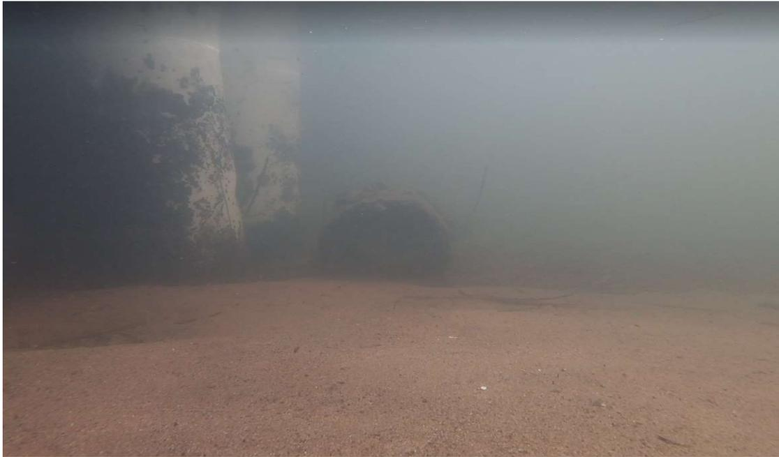
Photo 19: Seabed adjacent to southern jetty - fallen timber pylon visible
