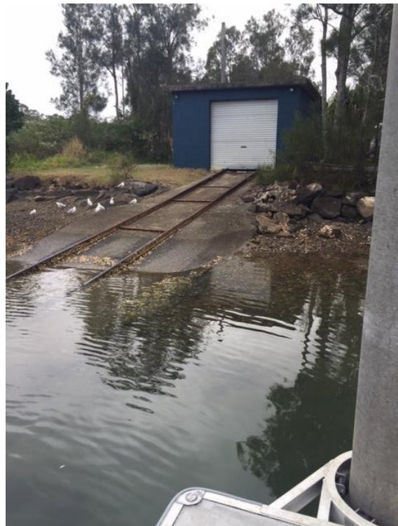
Emergency Services Slipway beside New Pontoon
