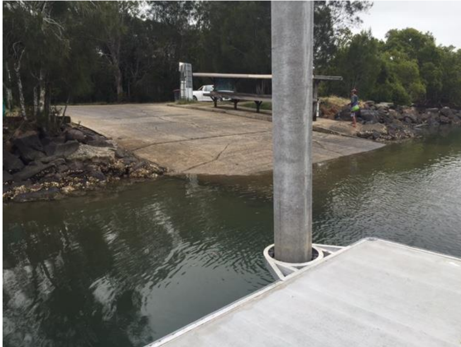
Existing River Ramp
