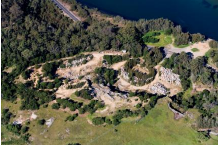
Aerial view of Quarry
