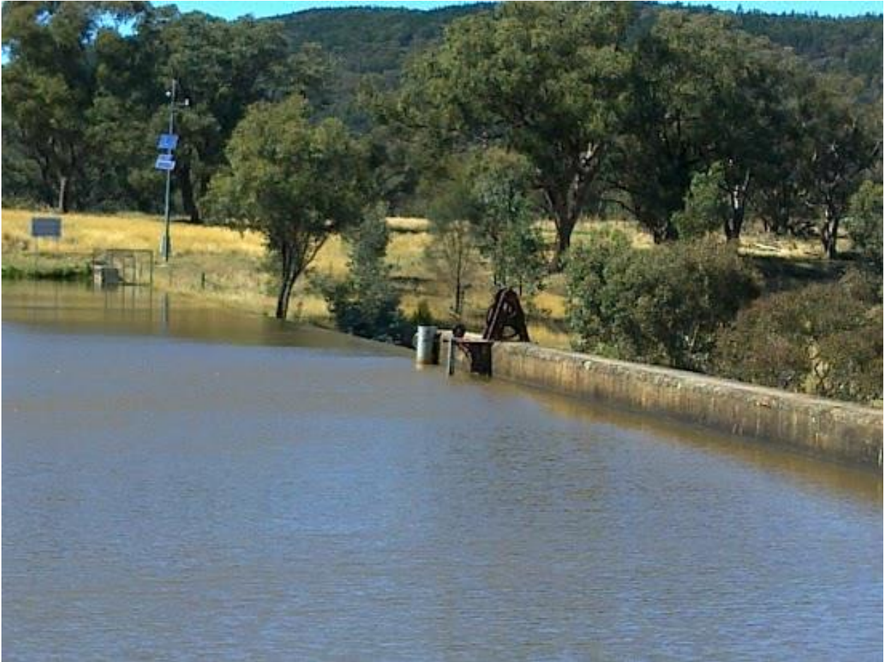
Figure 3 – Bethungara Dam - top of wall
