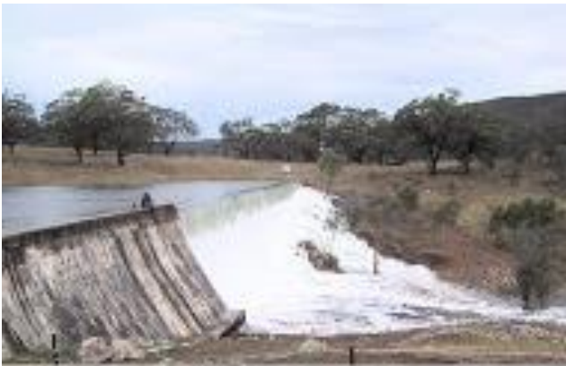
Figure 2 – Bethungara Dam during the 2003 flood
