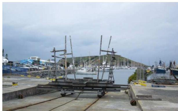
Coffs Harbour small slipway
