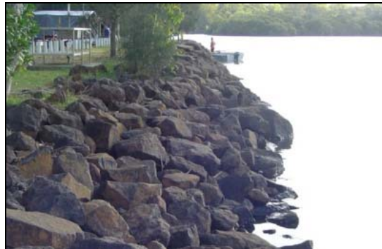
Plate 2.1 Example of a rock revetment seawall at Ferry Reserve Caravan Park
