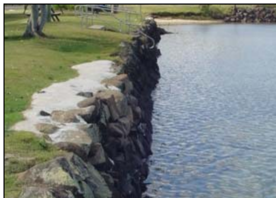
Plate 2.2 Example of a block seawall north of Terrace Reserve Caravan Park
