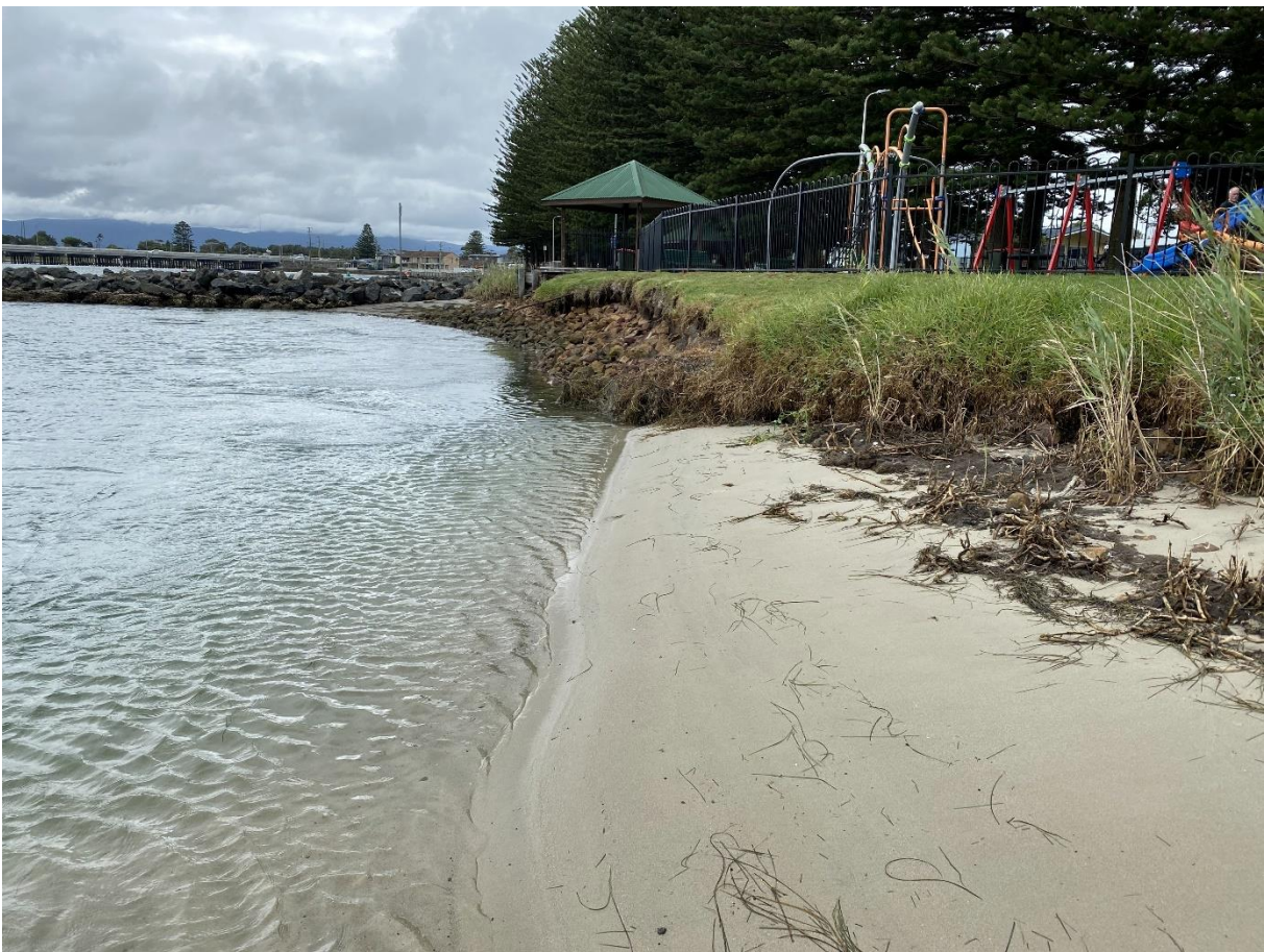
Figure 2.3 Erosion along the Windang foreshore immediately downstream of the groyne
