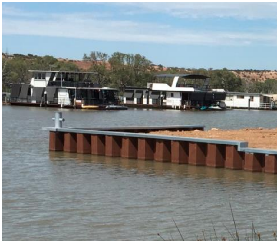
Figure 5.1 Example vertical steel sheet pile revetment
