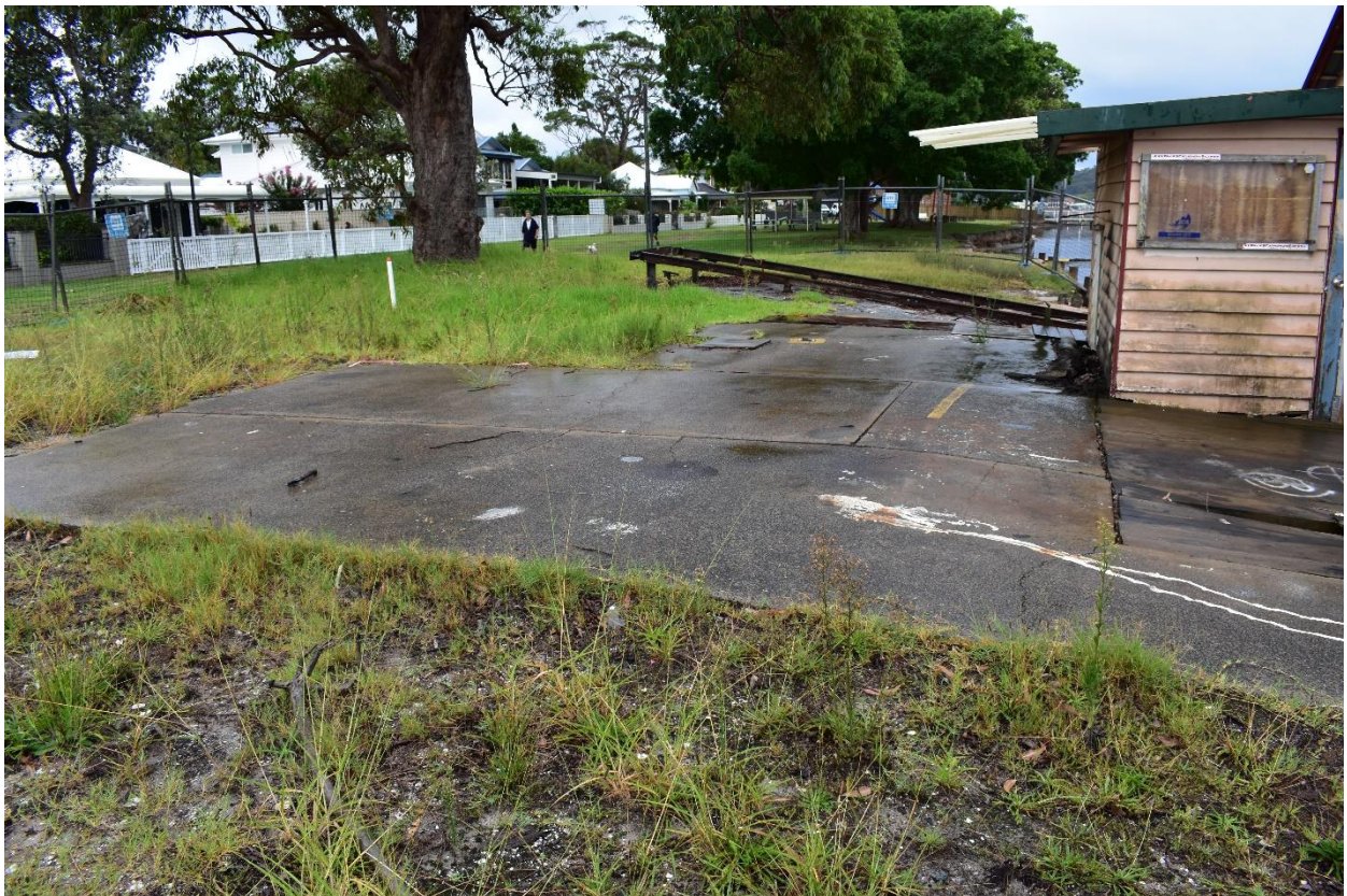
Figure 1.12 – Concrete installed over the underground fuel tanks, looking north along reserve.
