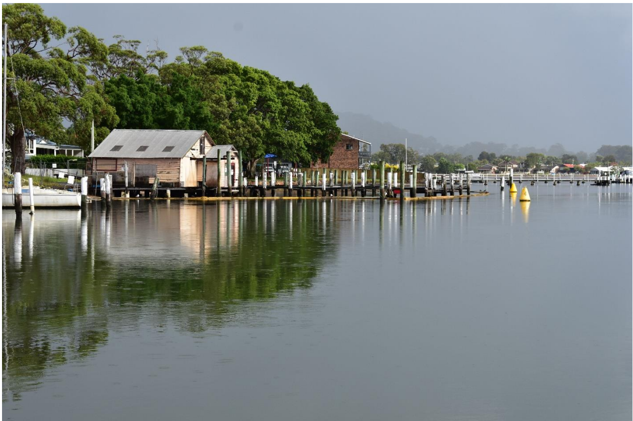
Figure 1.8 – Looking north to the Empire Bay Boat Shed showing jetties and floating silt curtain installed by Crown Land to contain debris.
