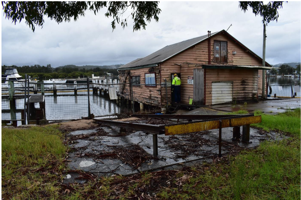
Figure 1.9 –Northern and western elevations with slipway rails in foreground.
