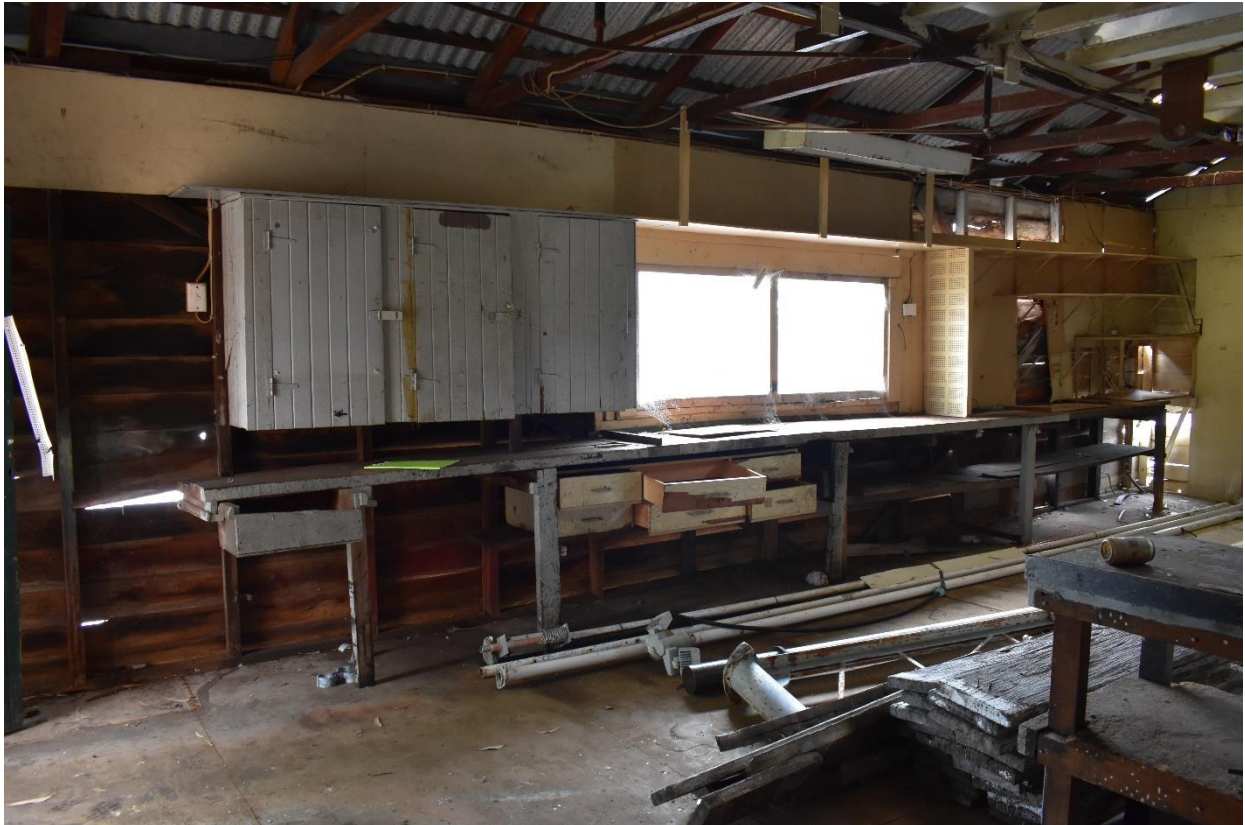
Figure 1.20 – Internal view of the northern elevation with fixed timber window.
