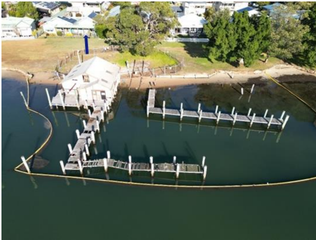
Figure 1.16 – Aerial view showing the jetties and Crown Reserve with the former Davis and Settree General Store shown at blue arrow. Image by Catalyst Consulting
