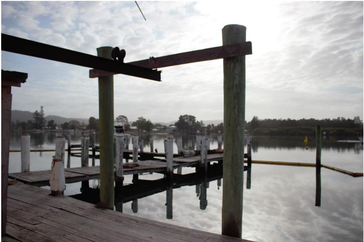
Figure 1.26 – Landing on eastern elevation of boat shed with uprights to support gantry – a modification dating to the 1980s. Beyond are jetties dating to the 1980s.
