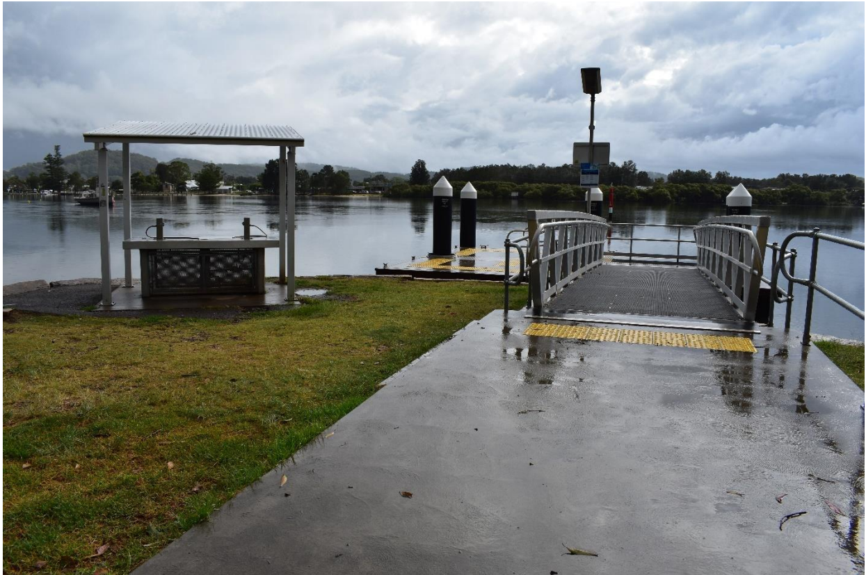
Figure 1.33 – Empire Bay public wharf.
