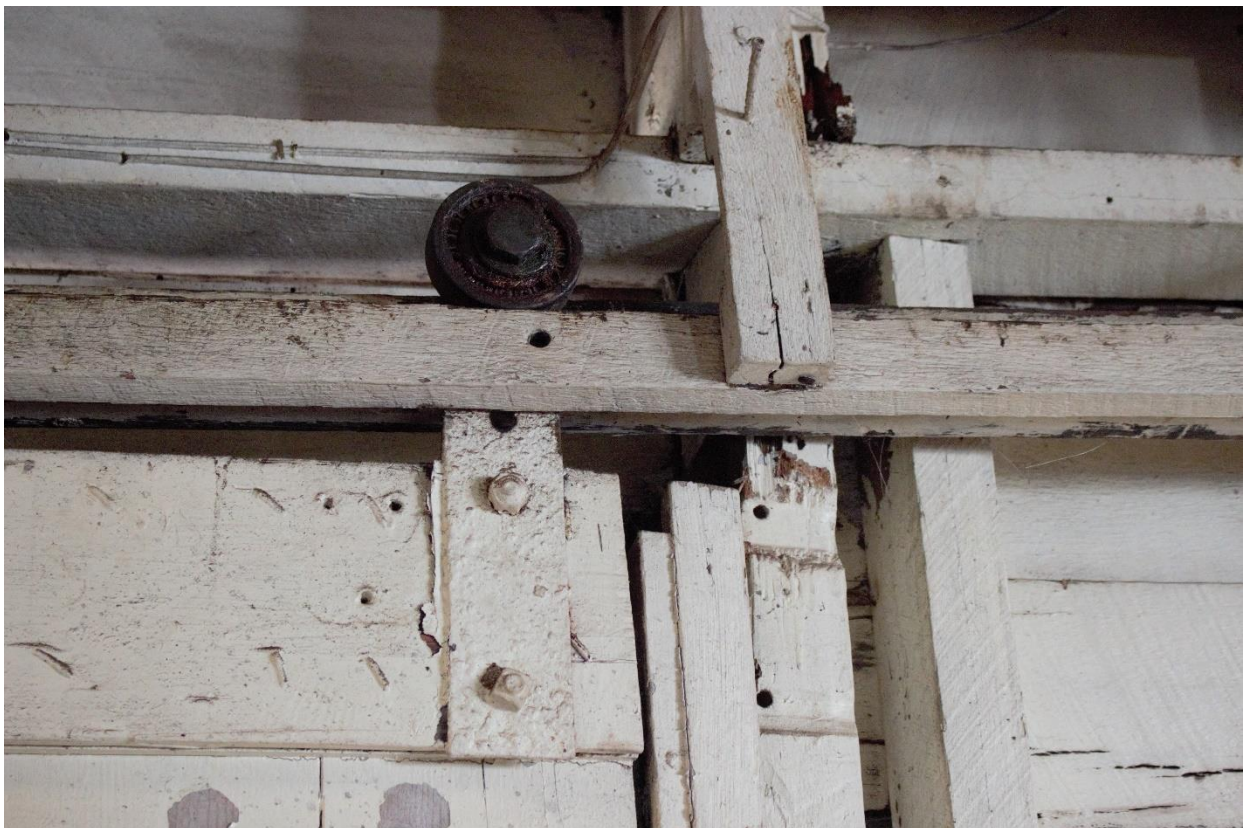
Figure 1.24 – Detail of roller mechanism on western sliding doors.
