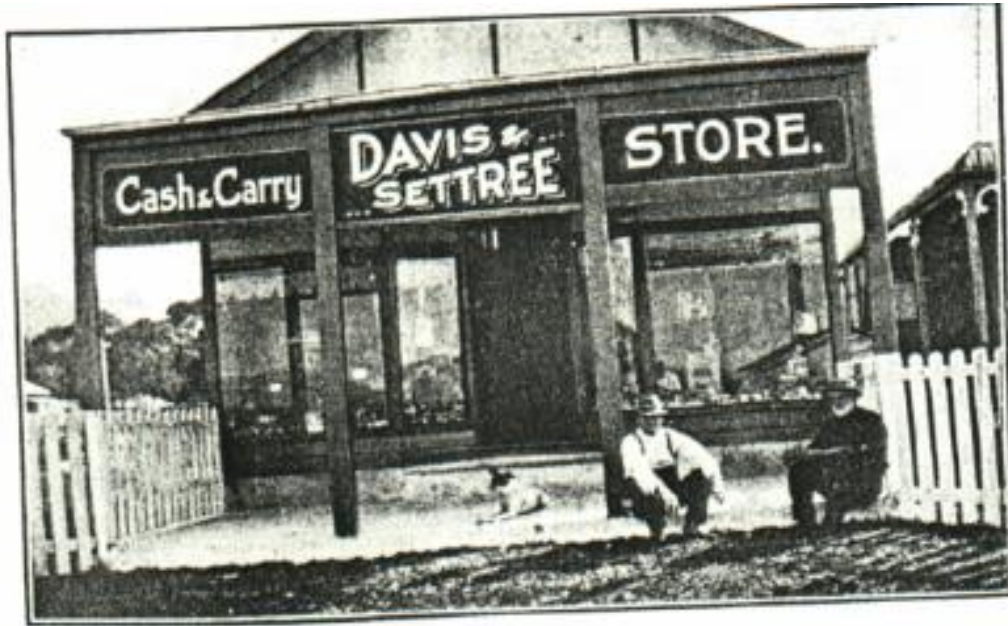
Figure 2.11 – The Davis and Settree Store c1930s located opposite the Empire Bay Boat Shed. Source: Central Coast Library Local History Collection.
