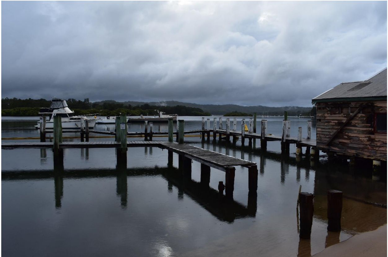
Figure 1.11 – Jetties on the northern elevation of the boat shed.
