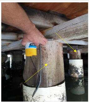
Photograph 17 shows another example of timber blocks placed upon the piers with no connection ties.
