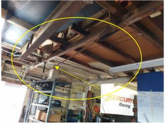
Photograph 34 shows the original ceiling frame has been modified with the addition of steel tension braces to underside of ceiling joists as a means of supporting the mezzanine loads.
