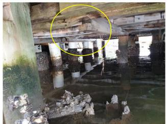
Photograph 25 shows a bearer with no support and furthermore breaking away from joist.
