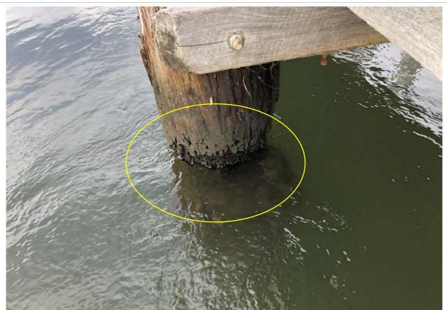
Photograph 70 shows an example of sectional loss as identified by structural engineer.
