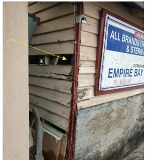
Photograph 42 shows the location where wind driven rain could affected the main switch board located behind this wall.
