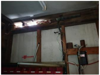
Photograph 43 shows where rusted roof sheeting above outdoor shower area is in fact allowing weather elements to enter a small storage area in the boatshed. Electrical wiring in close proximity.
