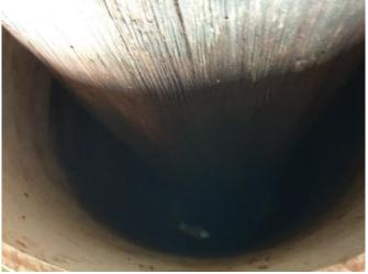
Photograph 24 shows example of many PVC shrouds are NOT filled with concrete (to encase decayed timber piers), even though that would be the anticipated purpose of these shrouds.
