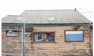
Photograph 48 shows the roof cladding above boat shed appears satisfactory.
