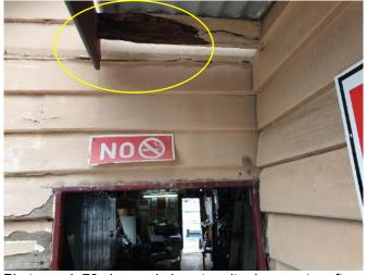
Photograph 79 shows obvious termite damage to rafters above door entry point.
