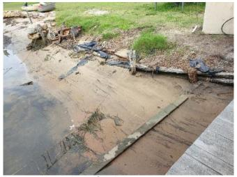
Photograph 63 shows Southern retaining wall in a collapsed / eroded state.
