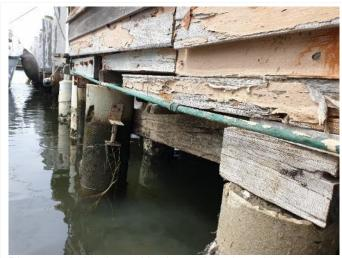
Photograph 18 shows Northern elevation with various timber blocks and 'add-ons' being utilised to support the subfloor structure.
