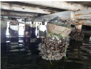
Photograph 21 shows a dilapidated cast concrete column that has been packed with concrete as means of supporting timber bearer. Again, inadequate repair type.
