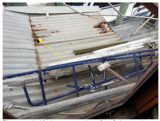
Photograph 46 shows corrosion of roof sheets above outdoor shower area.
