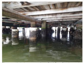
Photograph 1 shows overview of subfloor framing and supporting piers.
