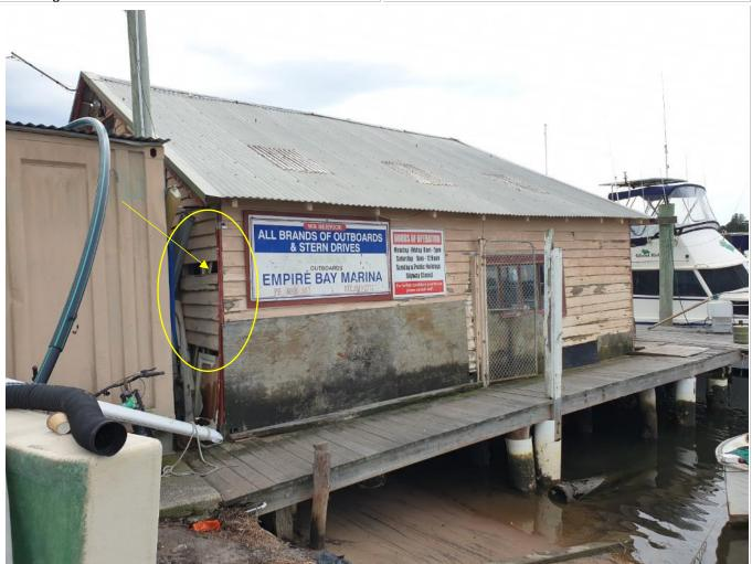
Photograph 40 shows missing weatherboards in which plywood now covers the area.
