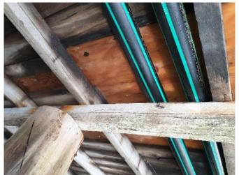
Photograph 20 shows missing portions of timber flooring, being covered over with plywood sheeting.
