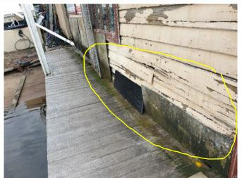
Photograph 41 shows weatherboards have fallen away and then the area has been covered over, but above that is more weatherboards which are loose.
