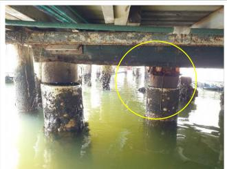
Photograph 8 shows another view point of where packing blocks are being placed upon piers.
