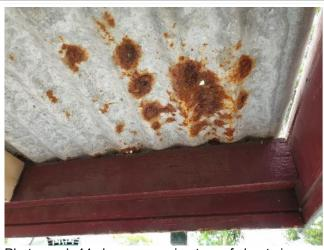
Photograph 44 shows corrosion to roof sheets is occurring.
