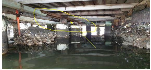
Photograph 11 shows steel C section placed in lieu where one would expect to see a timber bearer. Furthermore, there is timber packing blocks placed upon the piers to support the C section. An inadequate repair method. Again, ratchet straps are in use to tie supporting timber framing members together.
