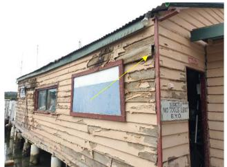
Photograph 39 shows loose weatherboard.
