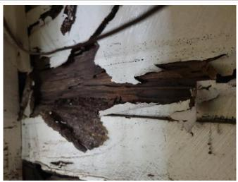
Photograph 75 shows termite damage to weatherboards.
