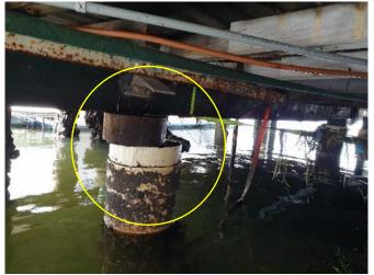
Photograph 7 shows where a pier continues to subside, with evidence of 'blocking' (packing) being placed upon each other. No visible tie downs to this location, meaning if the pier was to rotate, this section of floor would collapse.
