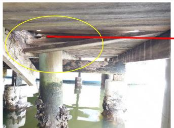
Photograph 14 shows the decking boards to Southern side that are collapsing due to lack of bearer support.
