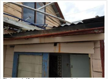
Photograph 45 shows corrosion to guttering.
