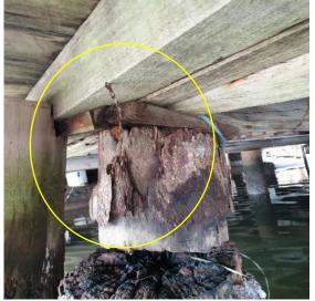
Photograph 22 shows timber wedges, blocking and lack of shoulder support for bearer.
