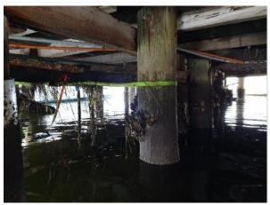
Photograph 2 shows an example of ratchet straps providing some form of support / tie -down / tension bracing to prevent separation in subfloor framing members.
