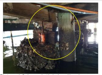
Photograph 5 shows a bottle jack positioned upon a very old pier that now supports the subfloor loading, again an inadequate method of repair. Note – there is 1x threaded rod that connects the green coloured pier to bearer, but that is again not an adequate means of supporting loading.
