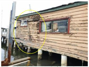
Photograph 38 shows an example of deteriorating weatherboards and failing fixings resulting in fallen cladding.
