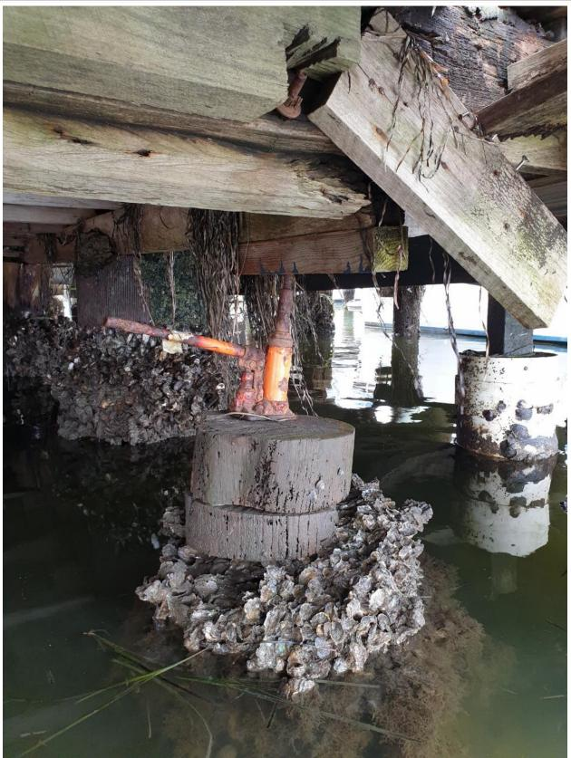
Photograph 13 shows a bottle jack, placed upon 2x timber packers, supporting 'structural' bearer and floor loads. It appears this has been in place for a 'long' period of time. Furthermore, we have other supporting timber framing members for decking that have fallen away.
