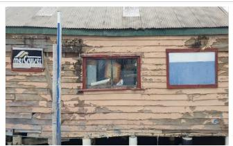
Photograph 61 shows an example where 2x windows have been covered over, along with centre window in a 'weathered' state.
