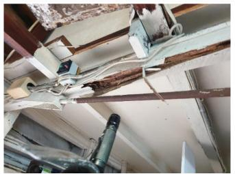
Photograph 77 shows termite damage ceiling joist which are in fact acting as mezzanine floor joists. Note - steel tension brace connected to subject timber. There's a heavy 'structural' reliance on this timber member.
