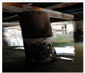
Photograph 10 shows another example of where a large section of timber has been placed on top of existing pier/ pile with no means of adequate strapping or hold down connecting that pier to bearer.
