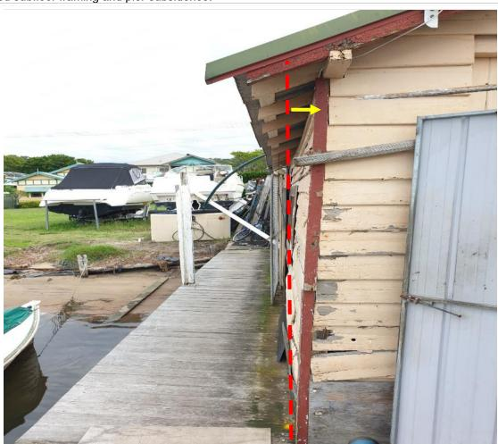
Photograph 31 shows the Eastern corner wall out of plumb, leaning to the right, again due to dilapidated subfloor and pier subsidence.
