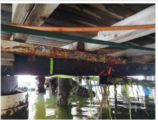
Photograph 4 shows ratchet straps securing a steel beam and old bearer / beam support. This is not a satisfactory repair method.
