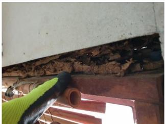
Photograph 76 shows termite damage to timber wall framing, located to loft / mezzanine area to Western wall.
