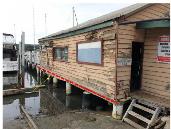
Photograph 30 shows an example of the deformation – sagging along bottom edge of external wall, due to dilapidated subfloor framing and pier subsidence.
