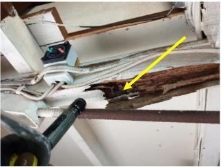
Photograph 78 shows large sectional loss to the structural timbers due to termite.
