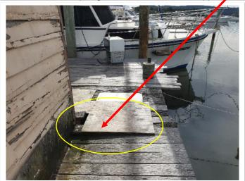
Photograph 16 shows the same location with a trip hazard present due to defective repair method.
