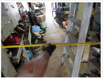
Photograph 60 shows general access width of 700mm wide at this location. Note all the stored items on the floor, which can pose a risk in the event of an emergency.
