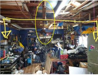
Photograph 35 shows the steel UB crane girder with drawing illustrating the distributed load points to wall framing. The issue with this is, if any live load is applied to the UB steel beam (i.e. engine lifting) then those loads are transferred down to subfloor and piles / piers which have serious structural defects.
