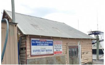
Photograph 47 shows the roof cladding above boat shed appears satisfactory.
