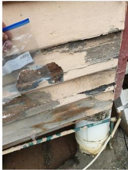
Photograph 67 shows an example of peeling paint being removed for testing.
