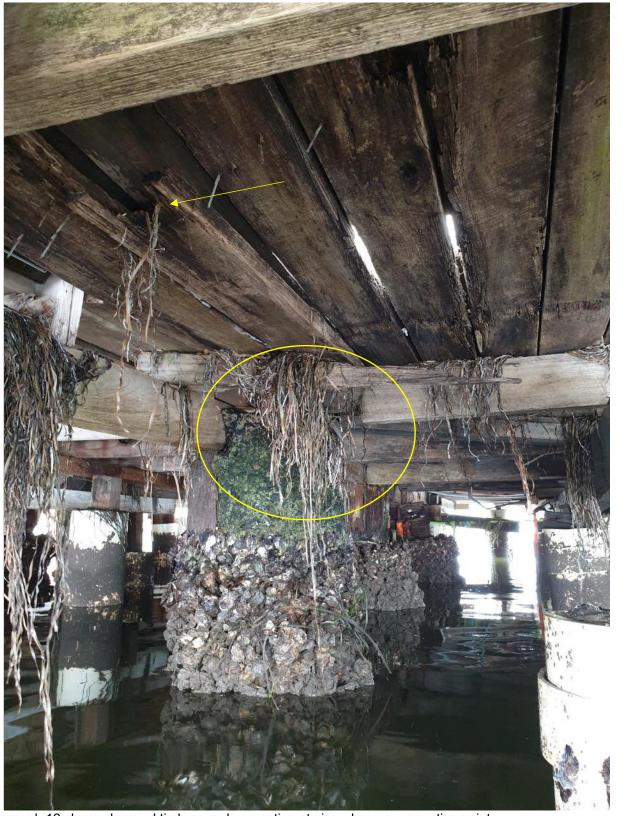
Photograph 12 shows decayed timbers and separation at pier – bearer connection points.
