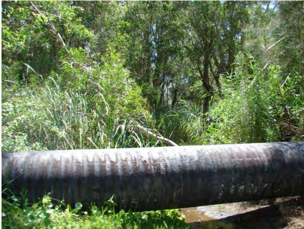
Photo 25: Raised sewage pipeline along the George Fire Trail
