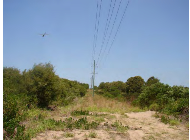
Photo 26: A high voltage electricity transmission line runs through the Park
