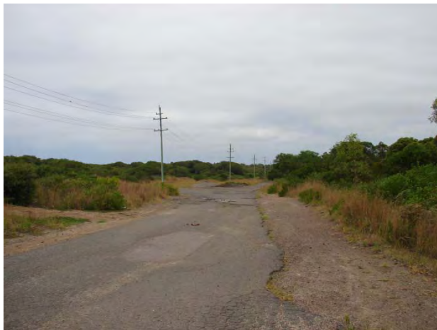
Photo 23: Kalaroo fire trail near the Kalaroo Road park entrance
