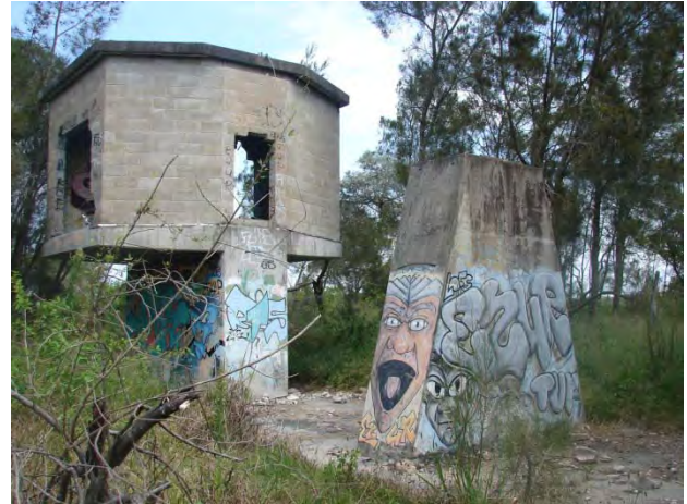
Photo 6: Decommissioned mining air shaft on Belmont Lagoon peninsula
