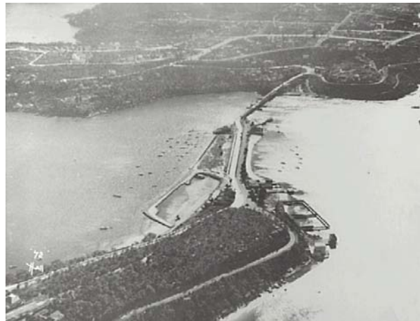
Figure 17: Construction of sea wall and Spit Reserve. Note the Spit Baths on the lower eastern side of the Spit. Mosman Municipal Library, http://www.mosman.nsw.gov.au/library
