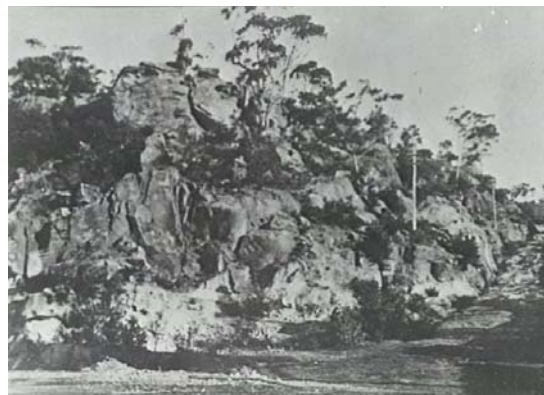
Figure 5: Natural condition of Parriwi Headland with the initial Upper Spit Road on the right, 1900. http://www.mosman.nsw.gov.au/library
