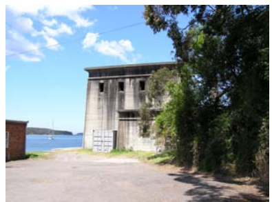
Sewer pumping station
