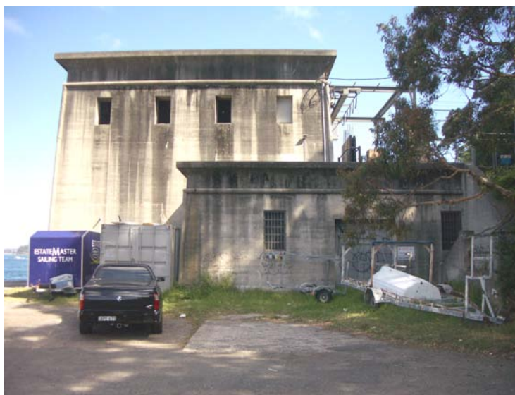
Figure 13: Middle Harbour Sewerage Syphon (Phillips Marler 2008).
